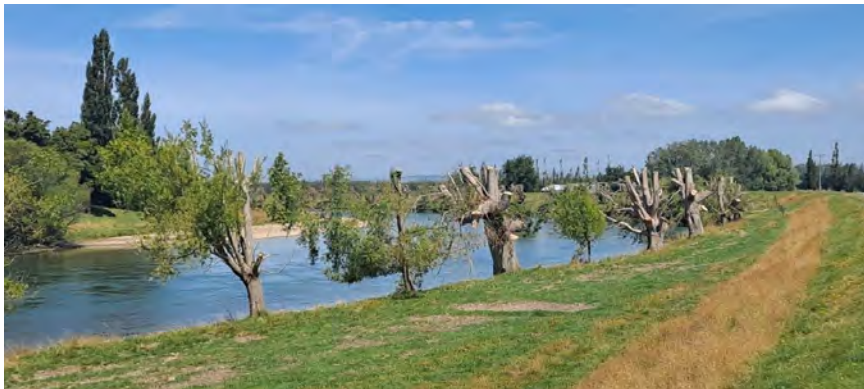
Figure 7 River Channel Tree defence assets, Lower Clutha River, February 2021
