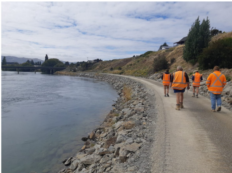
Figure 2 River channel asset, Albert Town (Clutha River/ Mata-Au) Rock Buttress flood repair works completed in February 2021.
