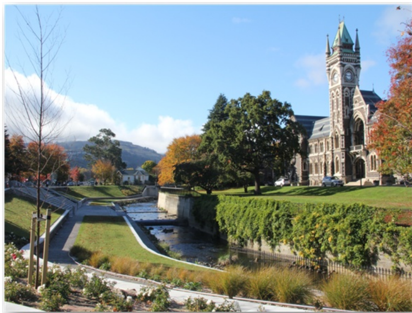
Figure 2: Leith Flood Protection Scheme at University of Otago Registry building
