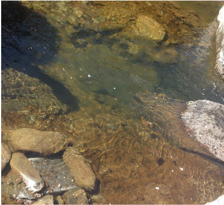
Photo 2.2: Bradfield Take – screened intake shown at bottom left
