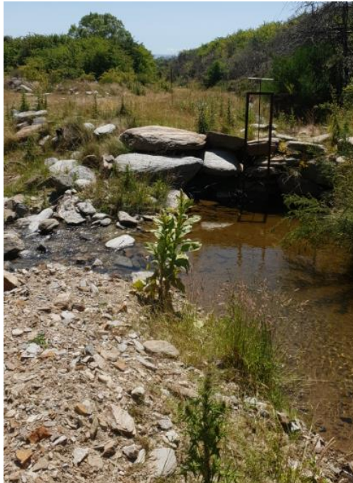
Photo 3.3: Herlihy Gorge Intake– Gate on race with by-wash back to Pigburn
