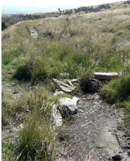
Photo 1.8: Re-take from Harpers Creek – standing upstream, looking downstream at re-take point (through pipe under rocks at right of photo).
