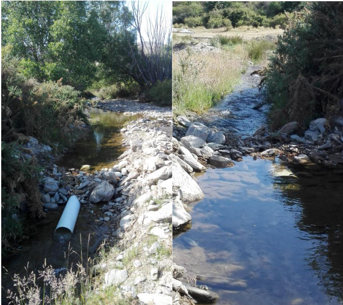
Photo 4.3: Weirs Point of take – looking down race at point of take, submerged pipe intake can be seen in middle of picture
