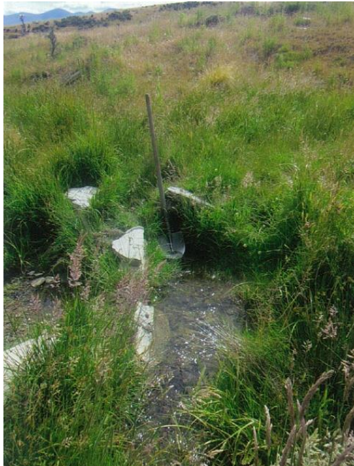
Photo 1.3: Shared Take - water race intake from Pigburn at intake pipe to the race.
