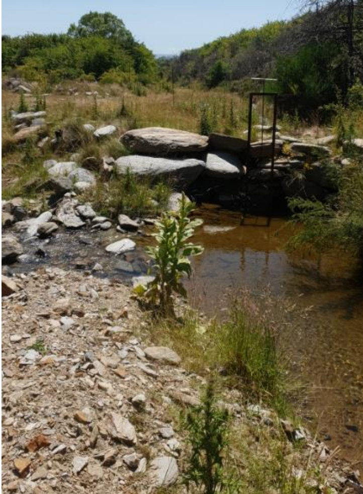
Figure 7: Herlihy Gorge intake, gate on race with by wash back to Pig Burn. (Source: Application).
