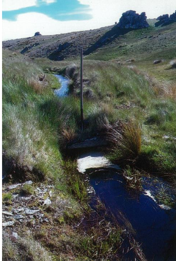
Figure 4: Shared take intake from Pig Burn and looking downstream at the race. (Source: Application)
