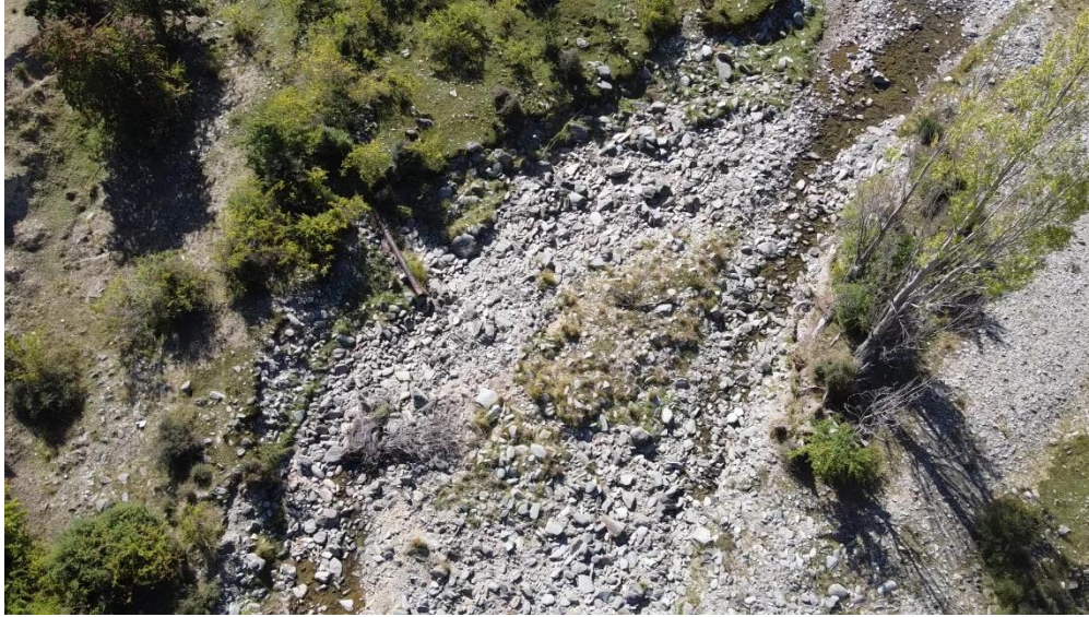
Figure 2 Aerial photograph of the upstream end of the upper drying reach of the Pig Burn on 18 March 2020. This is the area where flows became disconnected. Flow direction is from the bottom-left to the top-right of the frame.
