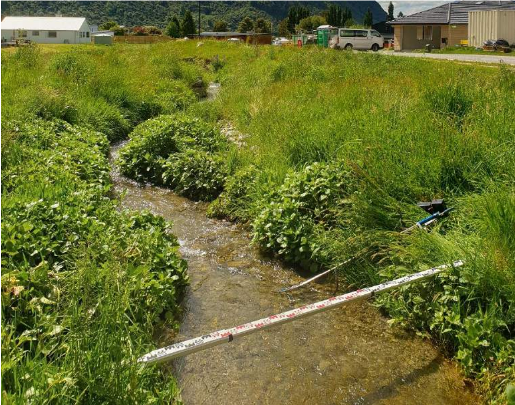
Figure 12: Downstream view of gauging section for KC 3.
