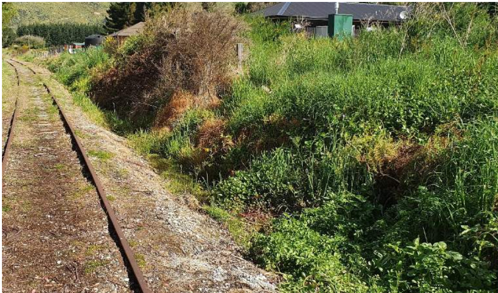
Figure 8: RD channel at RD 1.
