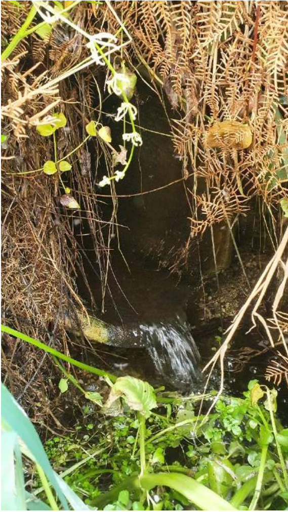
Figure 9: Pipe 5m below RD 1
