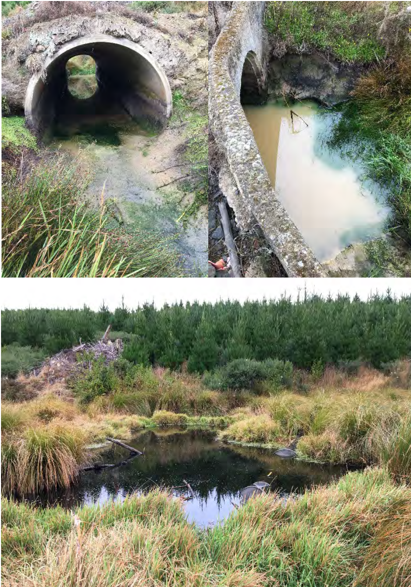
Figure 9. Otokia Creek tributary at the McLaren Gully Road culvert (top left: downstream of culvert; top right: upstream of culvert) and the large pond approx. 200-300 m downstream to the designation site, April 2021.
