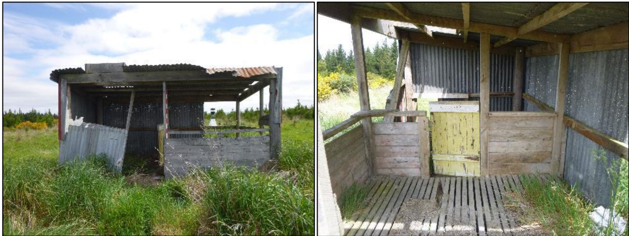
Figure 5-375-34 Site 7 Structure exterior (left) and interior (right).
