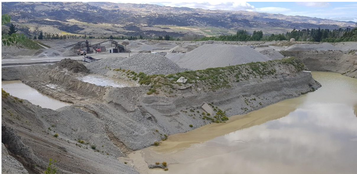
Figure 7. Photograph showing settling ponds that soak water to ground via main pond
