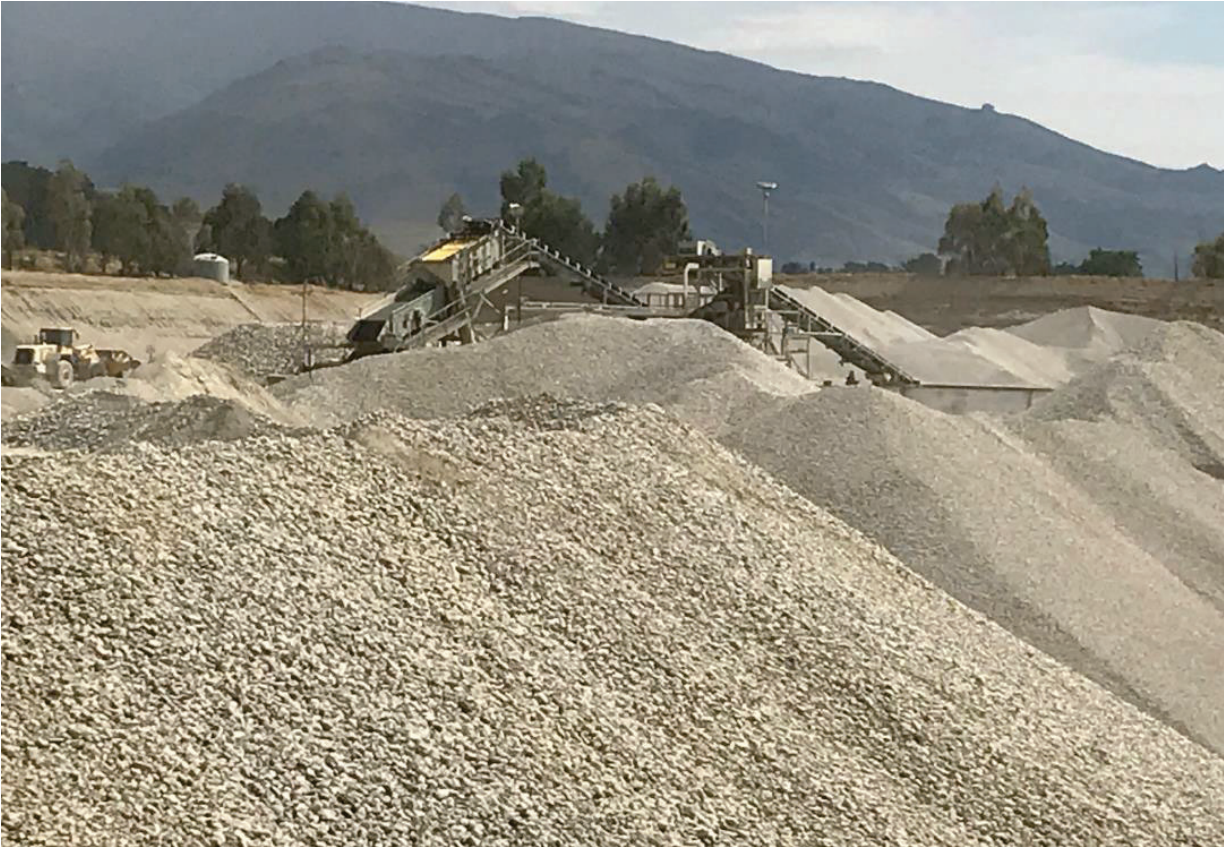
Figure 3-3 Photograph of screening and washing plant with washed aggregate in the foreground (21/1/2020)
