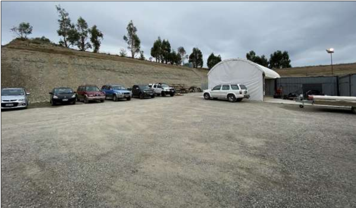
Figure 2: Quarry support facilities
