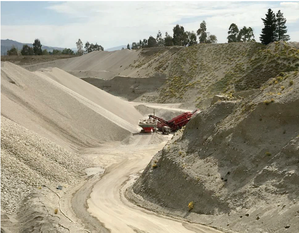
Figure 3-2 Photograph of mobile crushing plant operating on the quarry floor (21/1/2020).
