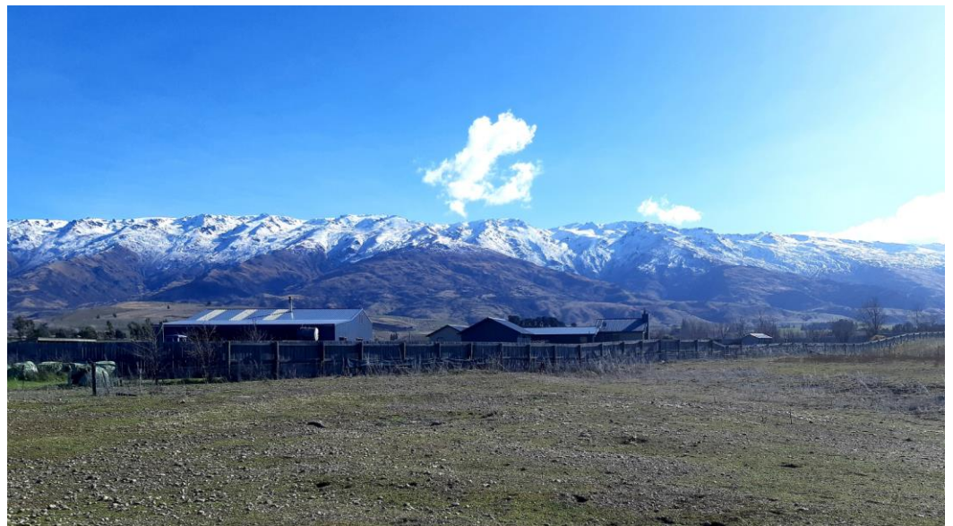
Figure 1: Dwelling at 1308 Luggate-Cromwell Road (to the right of photo). Note wooden fence along the boundary with the expansion land. Structure to left appears to be an outbuilding.
