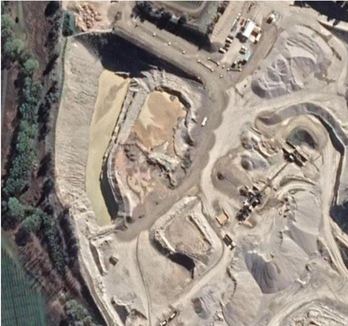
Figure 1: Aerial image of the soakage ponds with adjacent crushing plant
