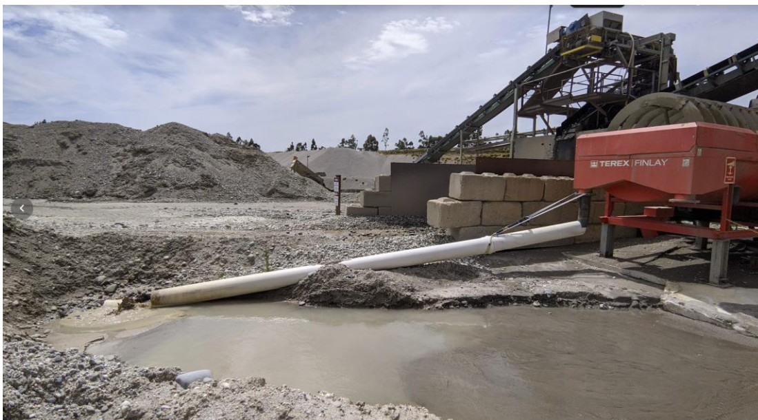
Figure 4b: Photos of the washing area and pipe to settling ponds
