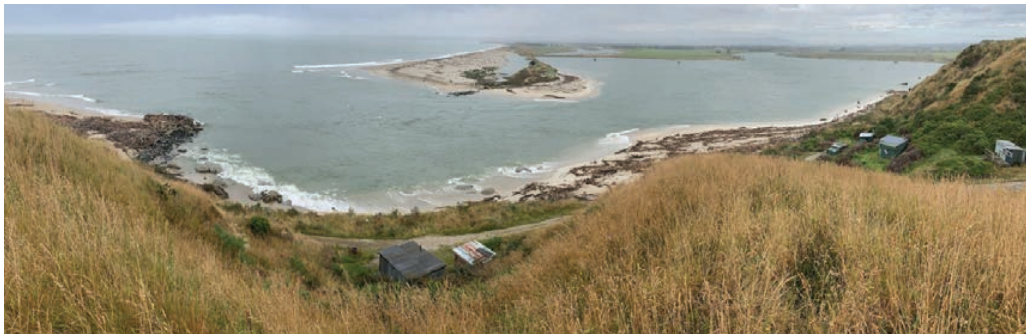
Figure 2.10: Matau River mouth looking south from Summer Hill showing the southern training line and the small northern rock groyne (Supplied by ORC, 2020).
