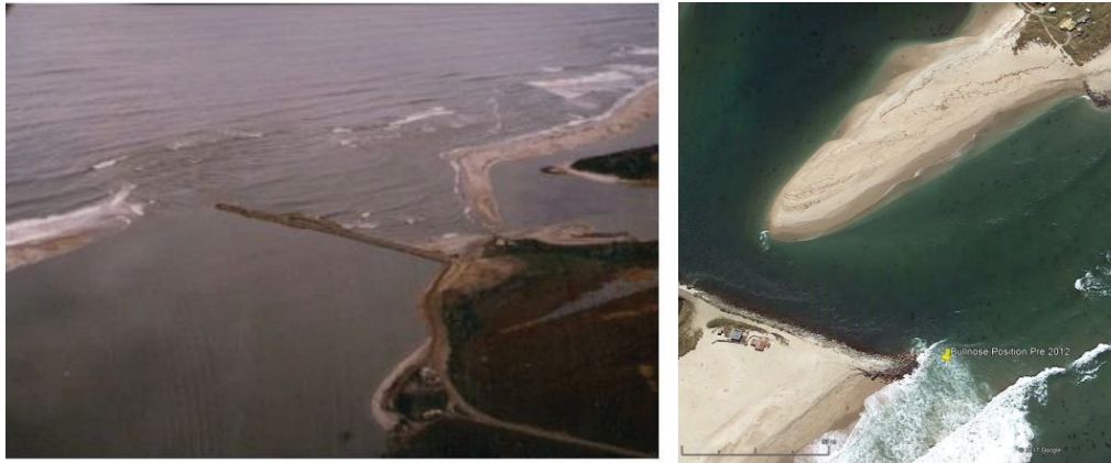
Figure 2.7: South training wall at the Koau River mouth. Photo A (left) - Under construction in May 1983; Photo B (right) - In 2016 from google earth imagery. Note the end of the northern wall can also be seen (Source: Bloor, 2017).
