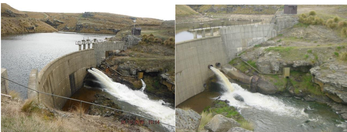
Figure 6: Onslow dam and outlets at relatively full lake levels (left) and lake levels 4.35 m below crest (right)
