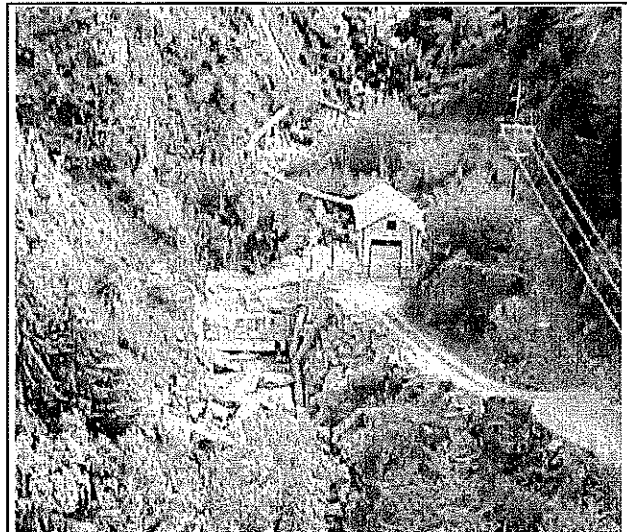
Upper Roaring Meg power house
