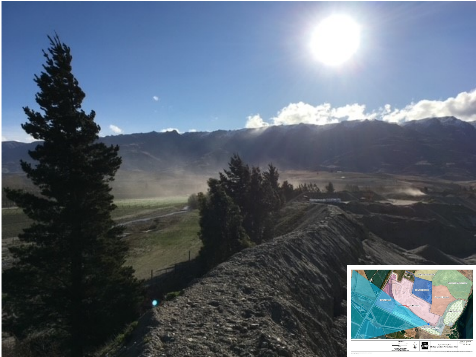
Figure 2: Picture taken on 31/08/2020 (looking west from the south-eastern corner of the quarry).
