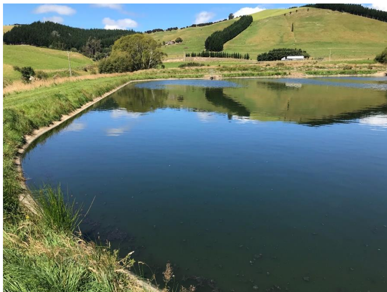
Figure 2: Waihola STP oxidation pond 2021 (Source: ORC Compliance Team)
