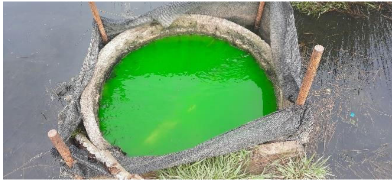
Figure 3.2.1 Dye released at the intake to the outfall pipe
