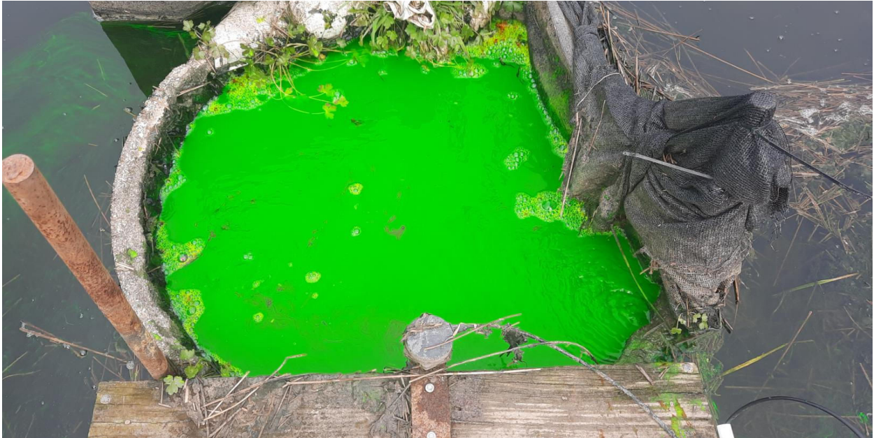
Figure 3.3.1 Dye released at the intake to the outfall pipe at 13:15 PM.
