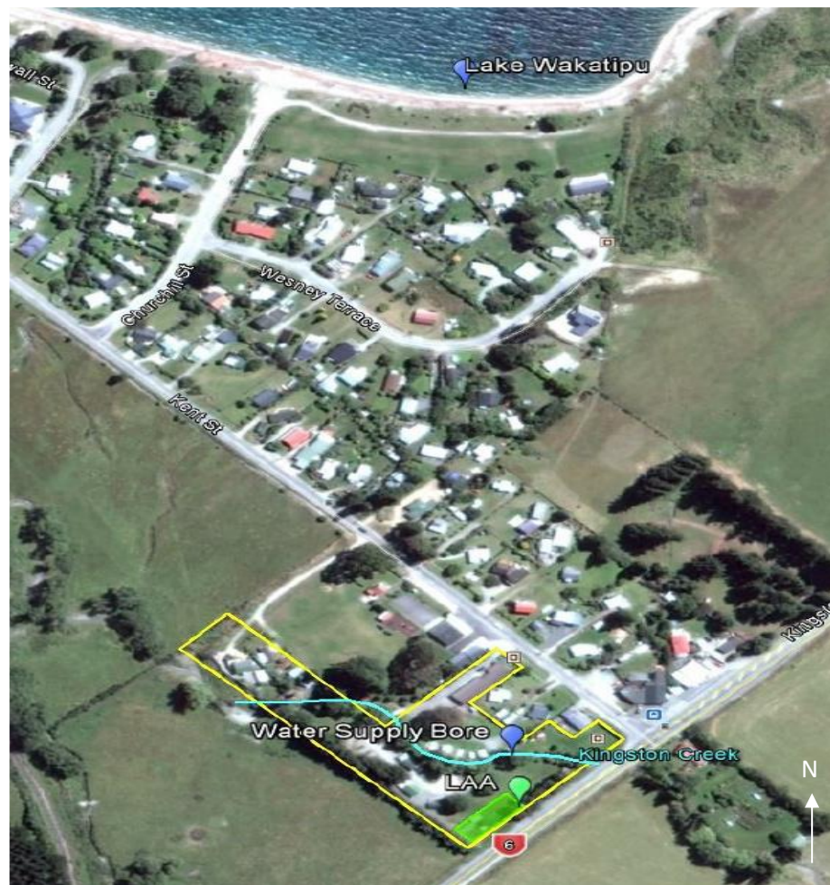
Figure 3: Kingston Holiday Park Limited Water Supply (Blue) and Disposal Field (Green Shaded area) (Source ORC S42 RM18052)
