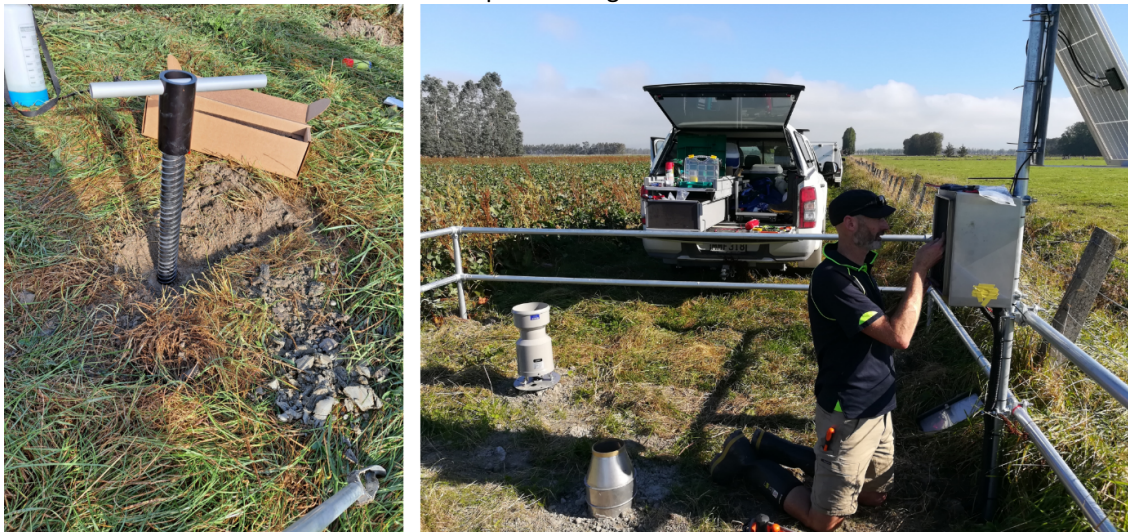
Fig. 14: Left: Soil moisture probe being installed. Right: Same site, showing the rain sensors and telemetry system (with Nick Boyens). The area is fenced off from stock and accidental damage by farming vehicles.
