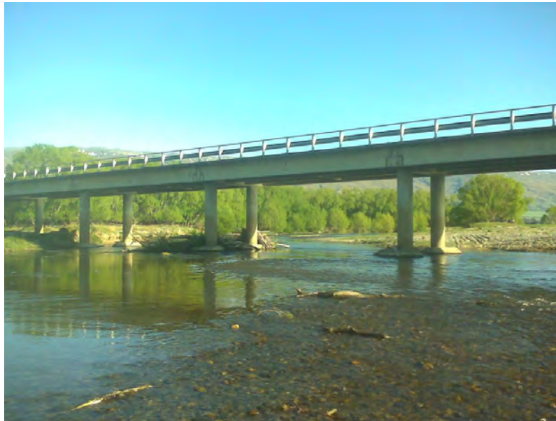
Figure 31. Cross-section ST7, looking upstream, November 2015
