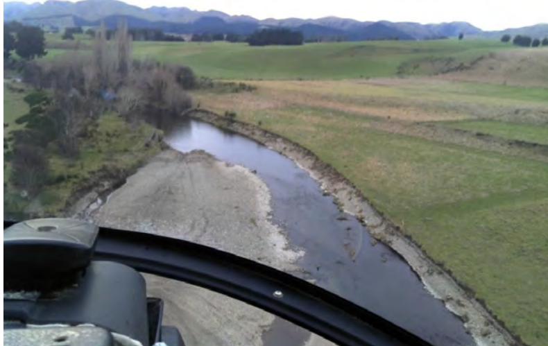
Figure 2. Example of changes in channel morphology, bank erosion downstream of Munro Road (looking upstream)
