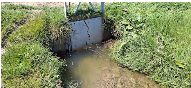
Figure 3 March Ck diversion sluice gate
