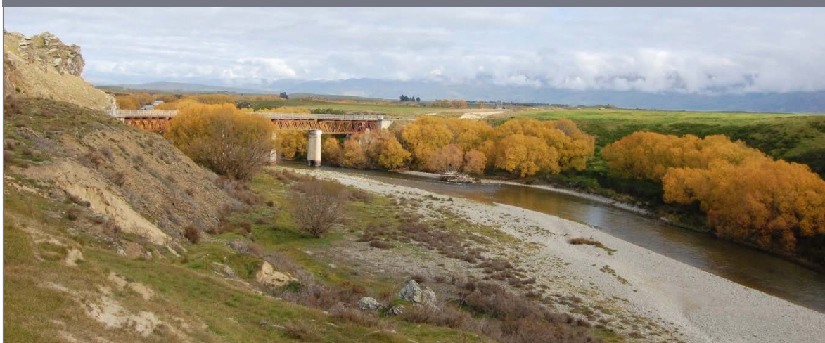
Manuherekia No. 1 Bridge. Otago Central Rail Trail east of Lauder
