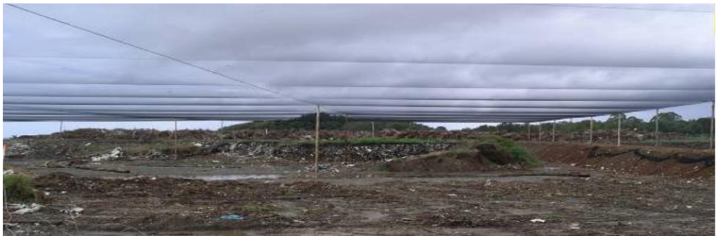
Figure 6. Ballina Landfill enclosed by a net allowing waste to be dumped in an area where access for birds was denied.
