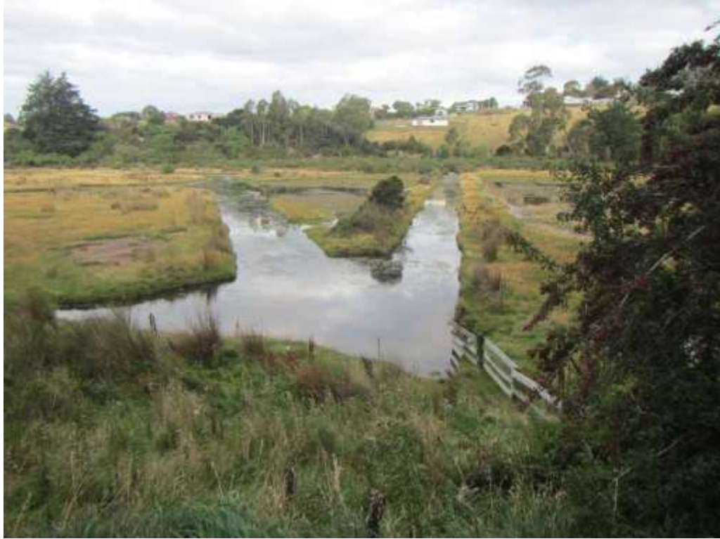
Plate 6: Excavated open water channels on the northern side of Lower Otokia Creek marsh.
