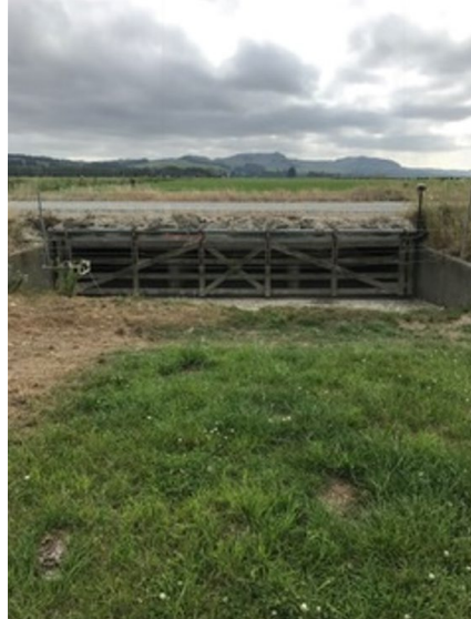
Figure 8: Eastern view of the Hilderthorpe Floodway Gray Road crossing
