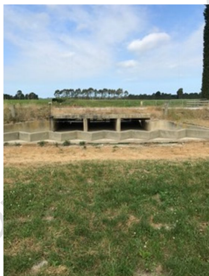
Figure 7: Western view of the Hilderthorpe Floodway Gray Road crossing
