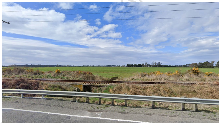
Figure 5: Hilderthorpe Floodway; view east from State highway 1 bridge.
