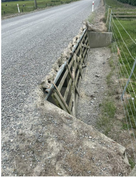
Figure 5: Hilderthorpe Floodway Culvert at Gray Road (downstream side)
