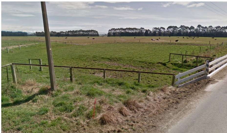
Figure 3: Hilderthorpe Floodway at Ferry Road (downstream). (Source: Google Streetview)
