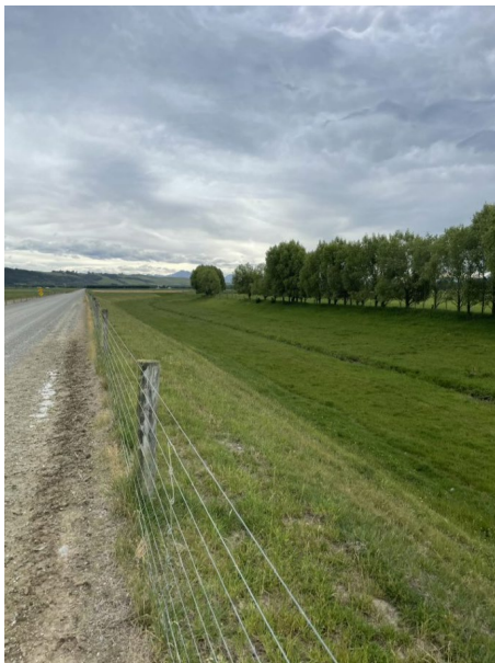
Figure 10: Henderson/Waikoura Floodway from Irvine Road (upstream)
