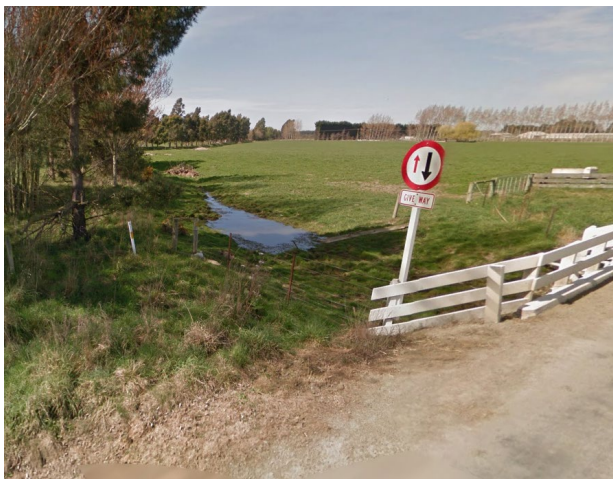
Figure 2: Hilderthorpe Floodway at Ferry Road (downstream). (Source: Google Streetview)
