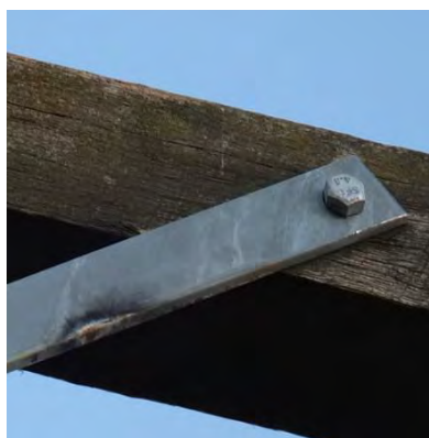
Fig. 45. Photograph (DSCF9361) above left identifies an arc mark to the lakeside metal stay arm on the upper section close to where it is secured to the wooden cross-arm with a double nut.
