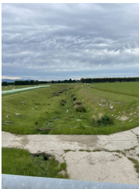
Figure 6: Waikoura Creek at State highway 83 (downstream)
