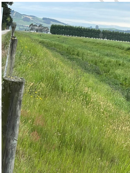
Figure 12: Henderson and Waikoura Creeks Floodway; viewed from opposite 550 Jardine Road, looking towards the south.
