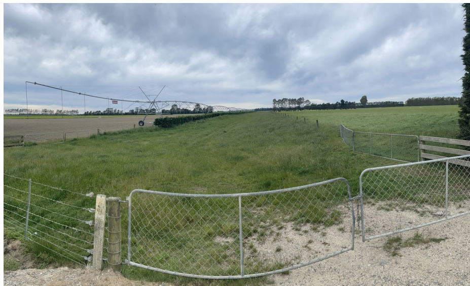
Figure 6: Hilderthorpe Floodway; view east from Gray Road crossing
