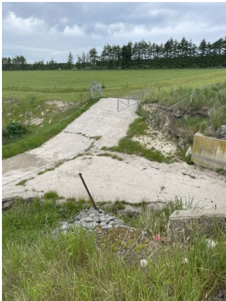
Figure 7: Waikoura Creek at State highway 83 (downstream)
