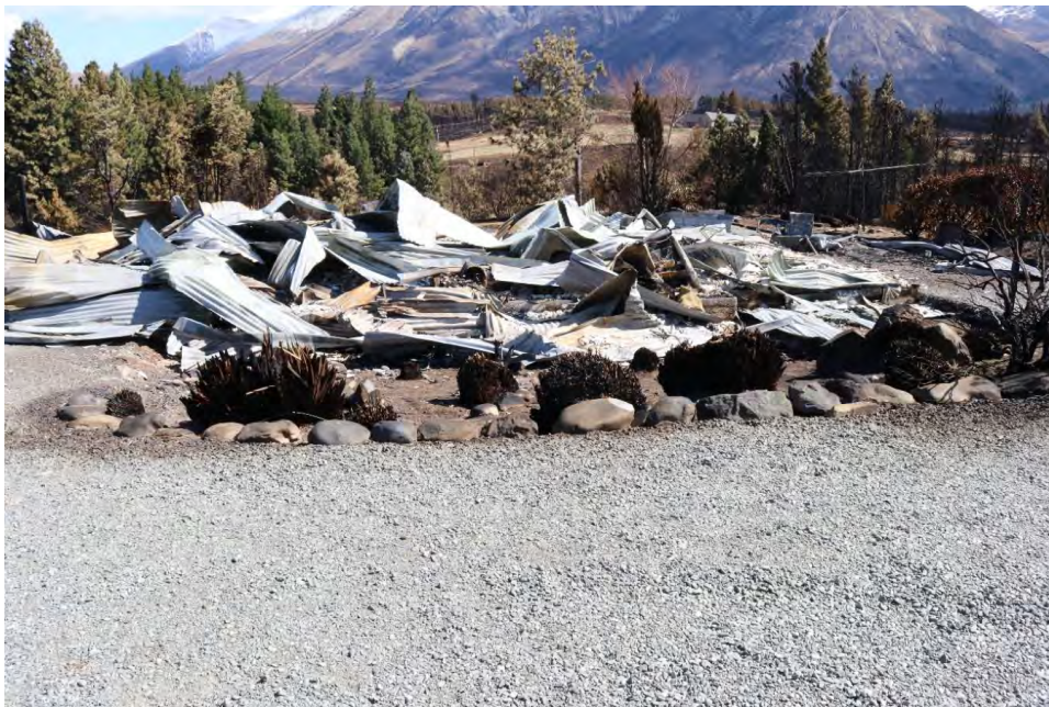
Fig. 19. An example of a building that was destroyed.
