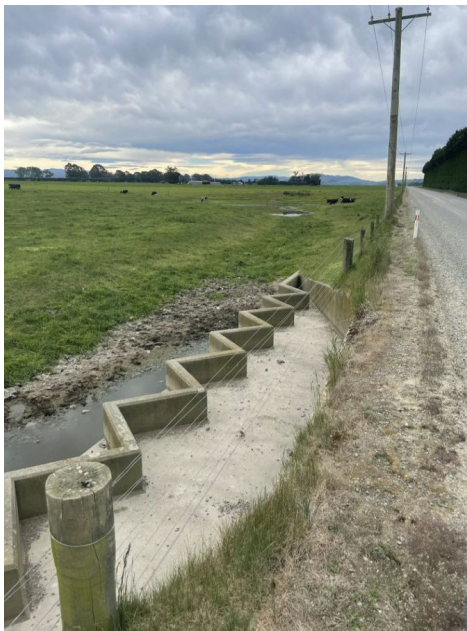
Figure 6: Hilderthorpe Floodway Culvert at Gray Road (upstream side)
