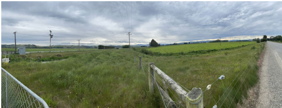
Figure 12: Henderson/Waikoura Floodway from intersection of Irvine and Jardine Road. Note irrigation canal to left of image
