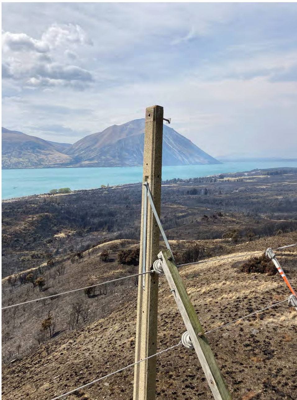
Fig. 56. Photograph (IMG_1712.JPG) above shows the lakeside metal stay arm hanging in the centre of the pole and the centre bolt that secured the wooden cross-arm to the pole has moved backwards but remains in the pole (note bolts have a single nut).
