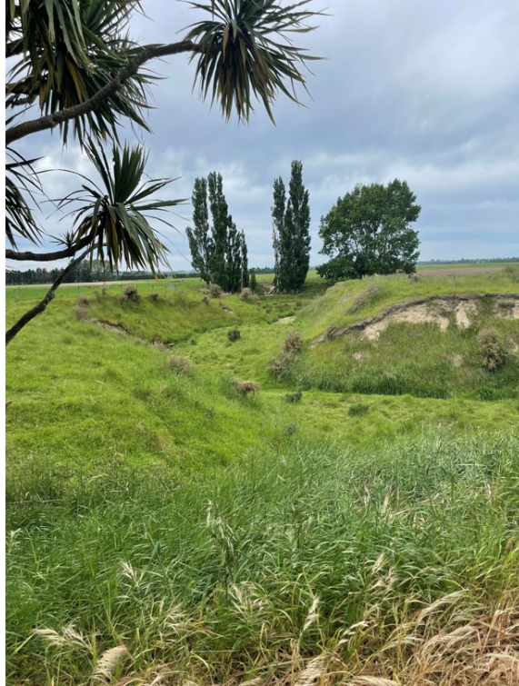
Figure 9: Henderson Creek Floodway, viewed from State highway 83 looking towards the north.
