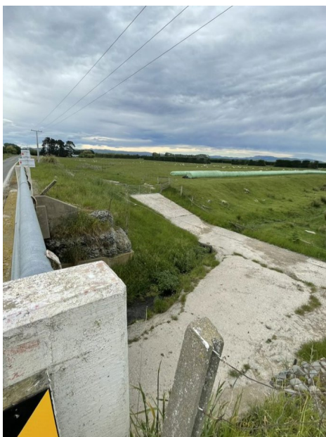
Figure 8: Waikoura Creek at State highway 83 (downstream)
