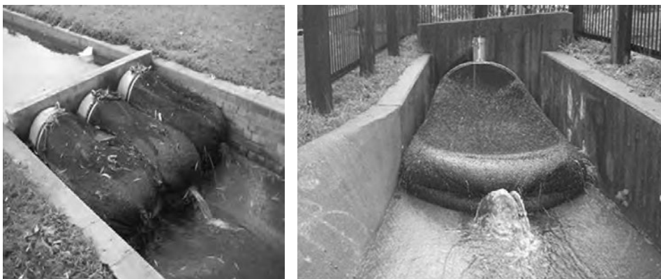
Figures 3&4 show the type of stormwater filters utilised in removing plastics that enter in significant waterways like the Otago Harbour.
