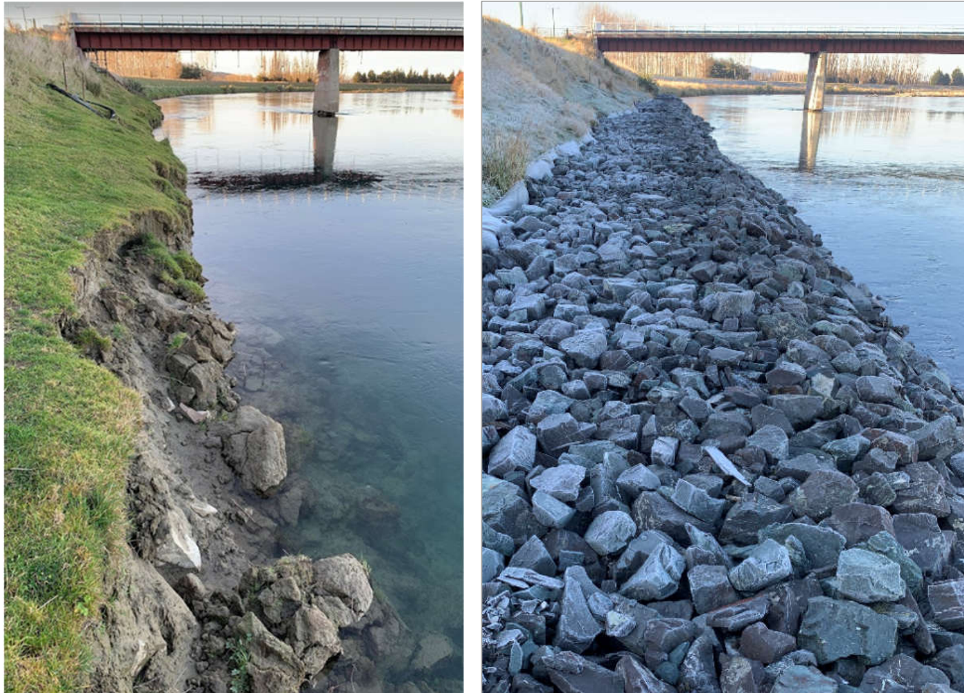
Figure 5. Riverbank Road floodbank at bridge near Stirling (LC21), before(left) and after (right) reshaping and vegetation stabilisation.
