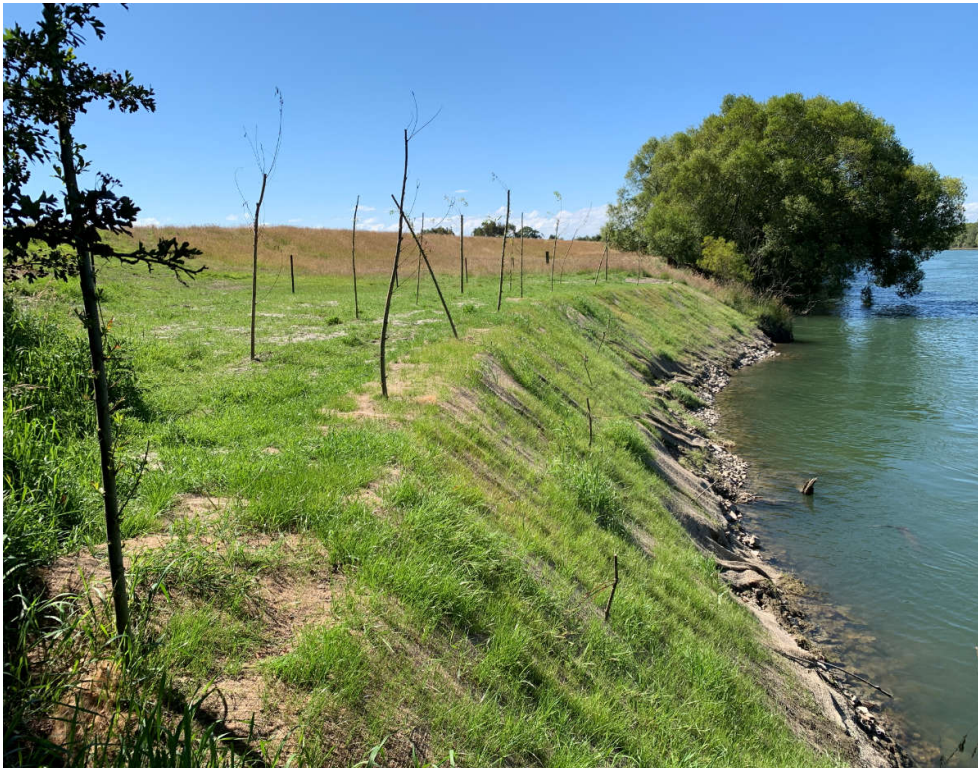
Figure 3. Riverbank Road (262 or LC18) floodbank before(above) and after (below) reshaping and vegetation stabilisation.
