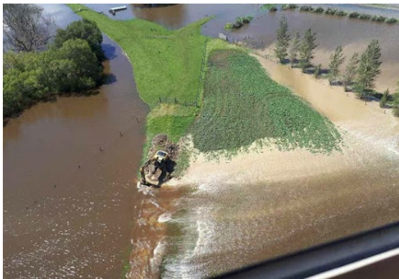
Figure 4. Excavating spillway during flood (5 February 2020).
