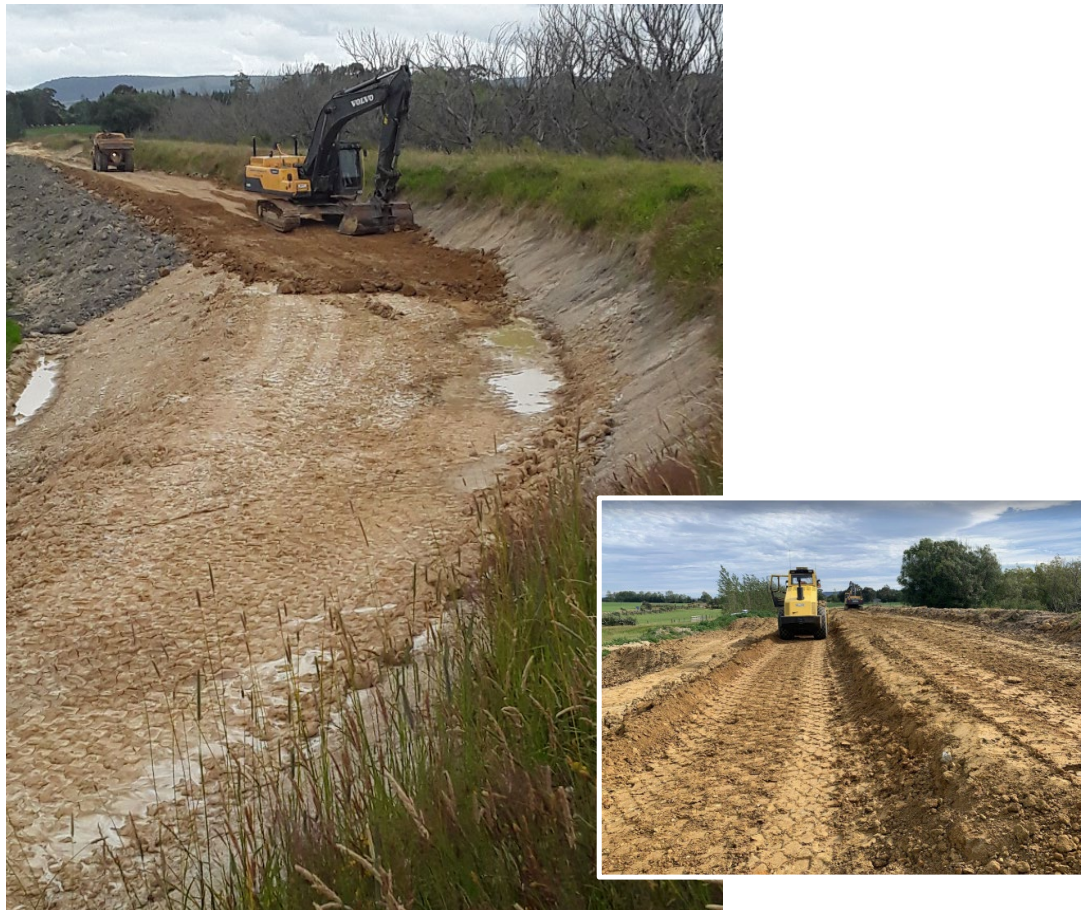
Figure 7. Repair of embankment toe
