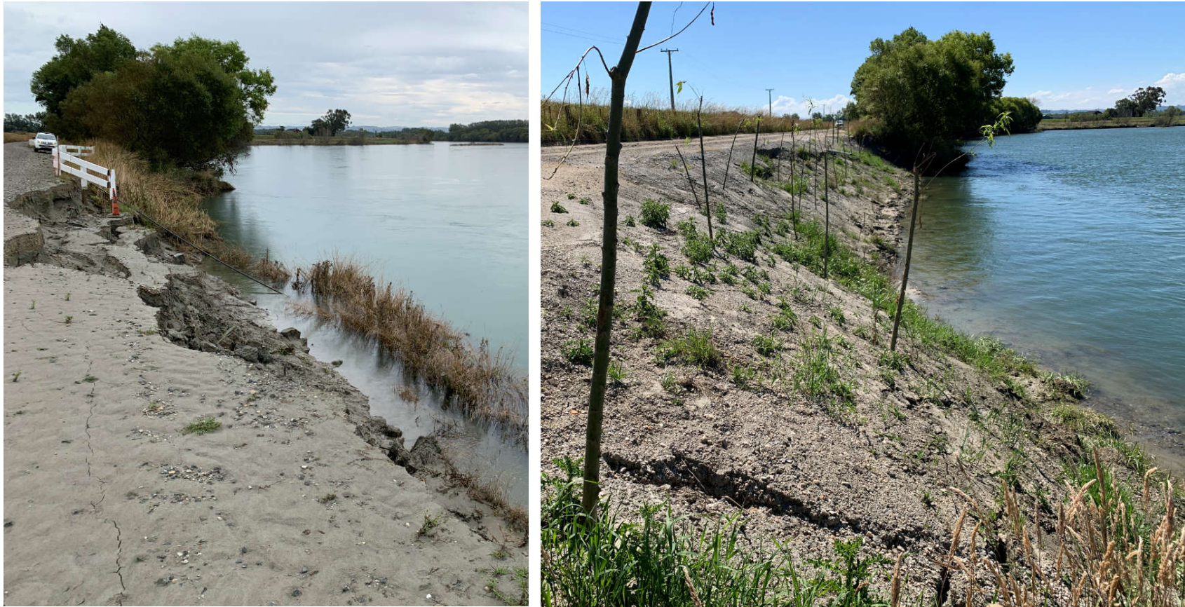
Figure 2. Riverbank Road at Renton Road (LC17) floodbank before and after reshaping and vegetation stabilisation.
