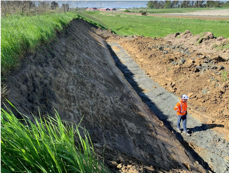
Figure 6. Repair of slumped section of embankment
