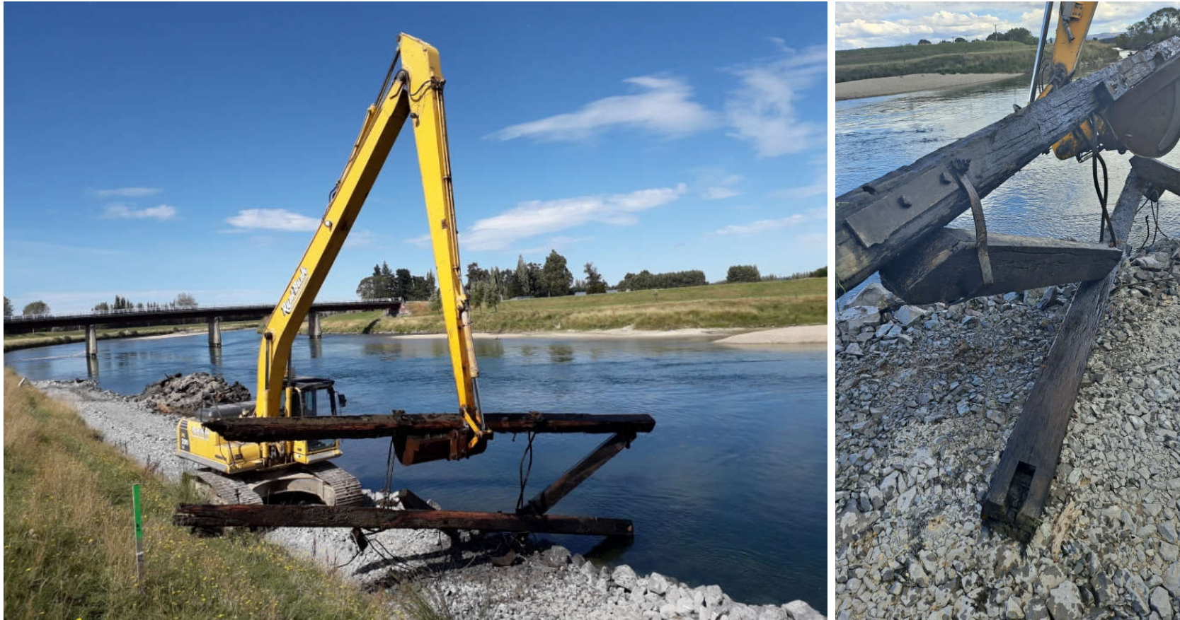
Figure 6. Discovery of historic (Pre-1900) bridge beams at Riverbank Road floodbank works at bridge near Stirling (LC21).
