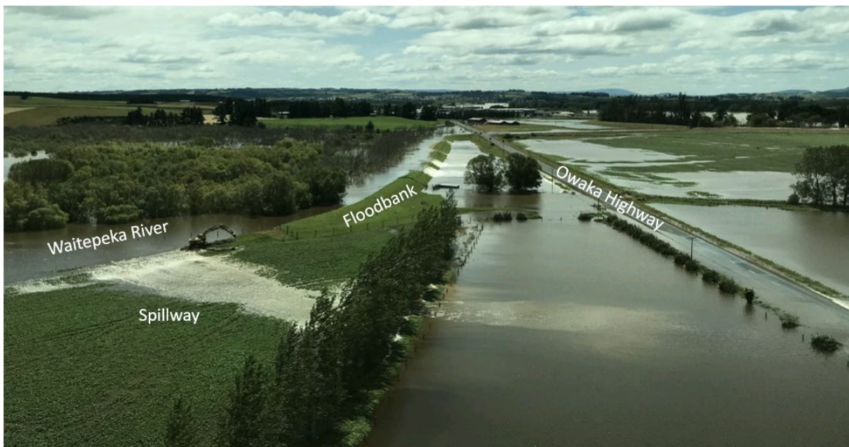
Figure 2. Waitepeka Floodbank during flooding. 5 February 2020.
