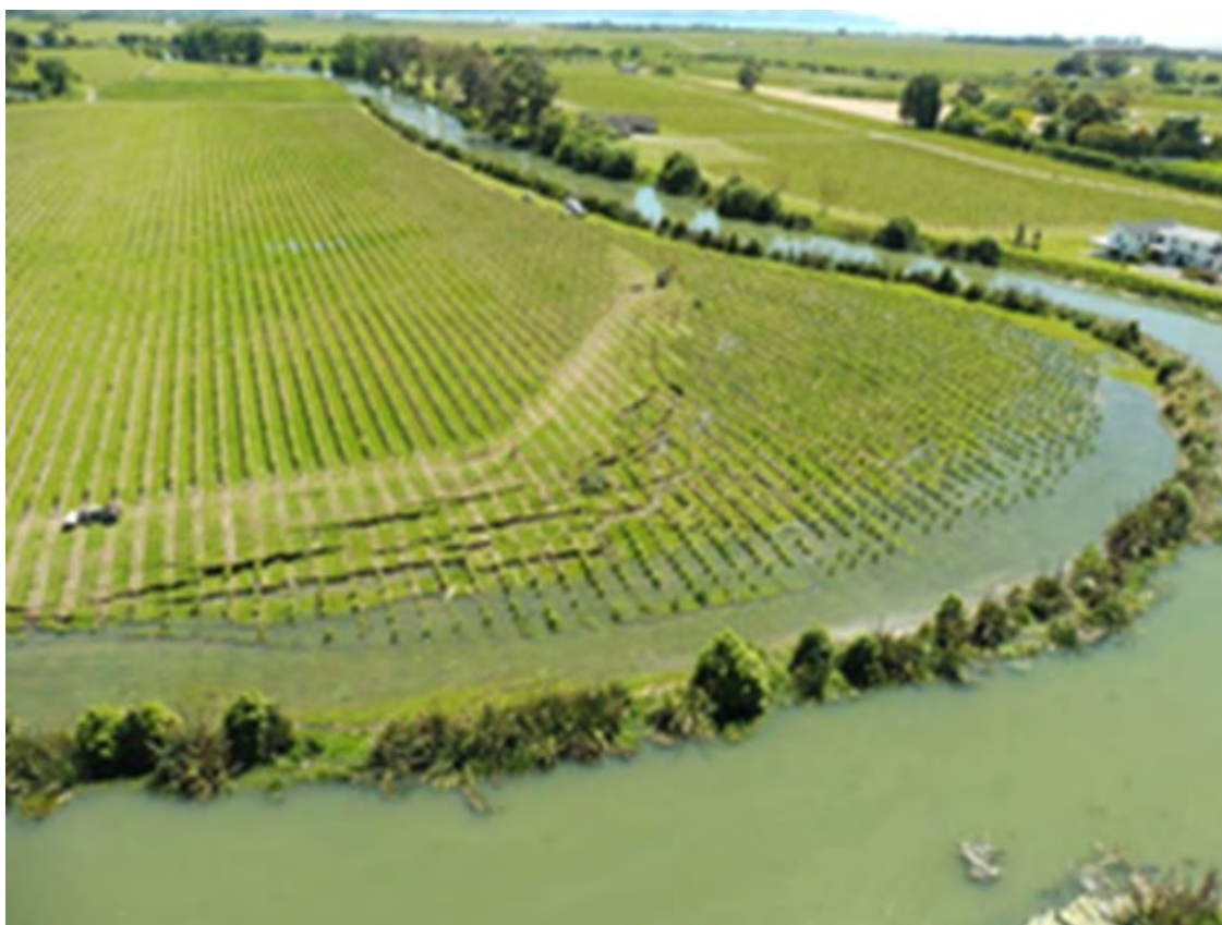
Figure B3 – Photo showing the lateral spreading that occurred in Blenheim at a vineyard along the Wairau River following the 2016 Kaikoura earthquake. The lateral spreading horizontal movement was approximately 3m and the vertical drop was approximately 1m (approx. 33% of the horizontal movement).
