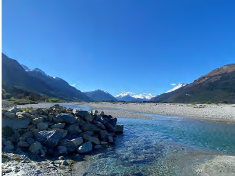
Example of a typical rock groyne constructed on the true right bank of the Dart River with significant scour on the downstream side of the groyne.
