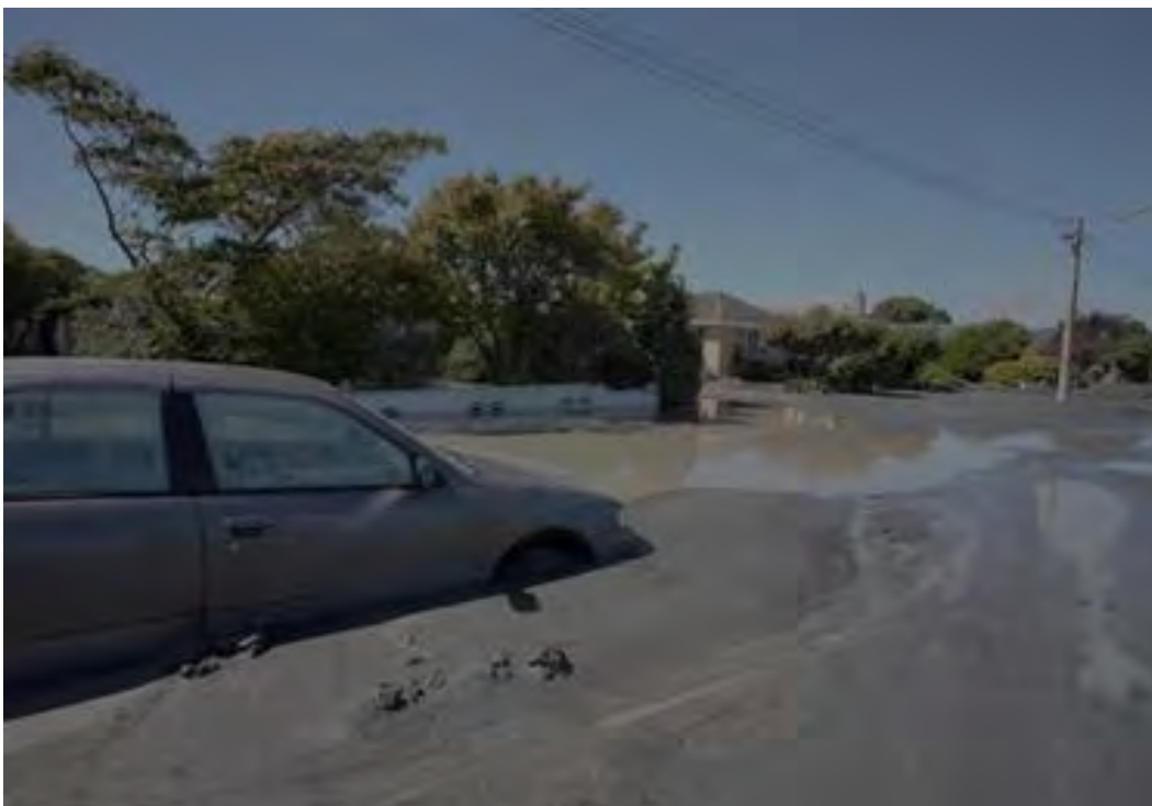
Figure B10 - Photo showing liquefaction in Christchurch following the 2011 Christchurch earthquake. Approximately 400 to 500mm of liquefaction ejecta inundated the roads.
