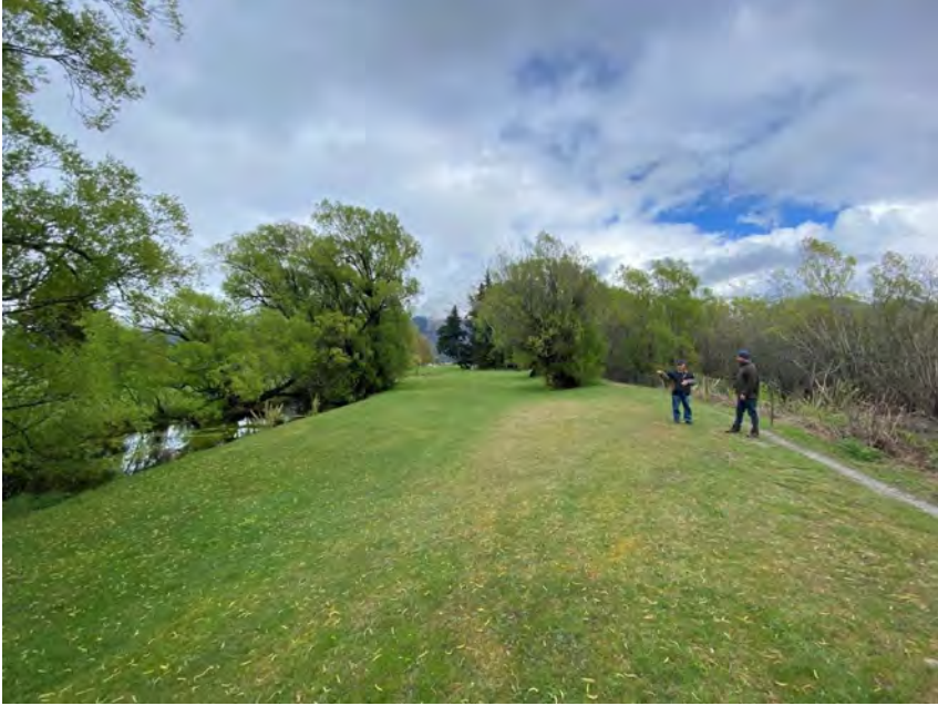
Photo of Glenorchy Stopbank adjacent to the Golf Course (overflow location)
