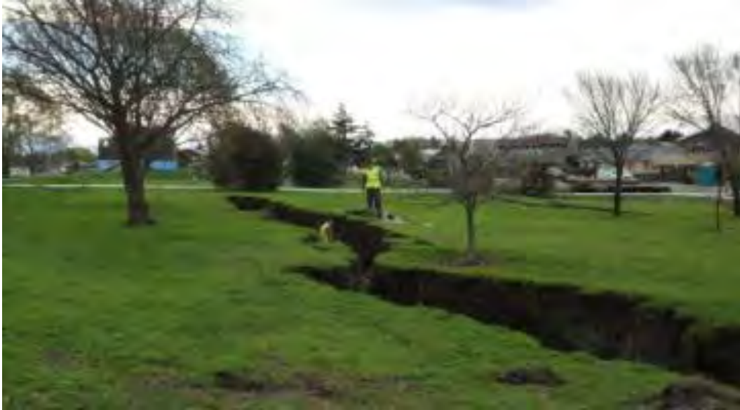
Figure B8 - Photo showing lateral spreading at Charles Steet, Kaiapoi following the 2010 Darfield earthquake. The total lateral spreading at this site was approximately 1.5m. Vertical offsets in the order of 300mm can also be seen in the photo (approx. 20% of the horizontal movement).
