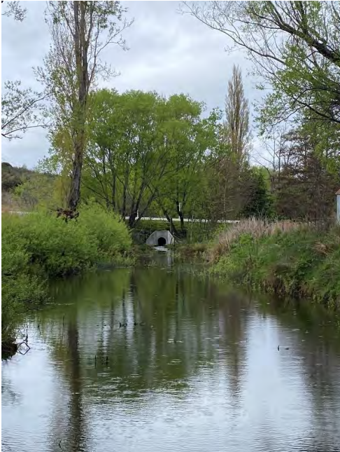
View of culvert under Glenorchy-Paradise Road
