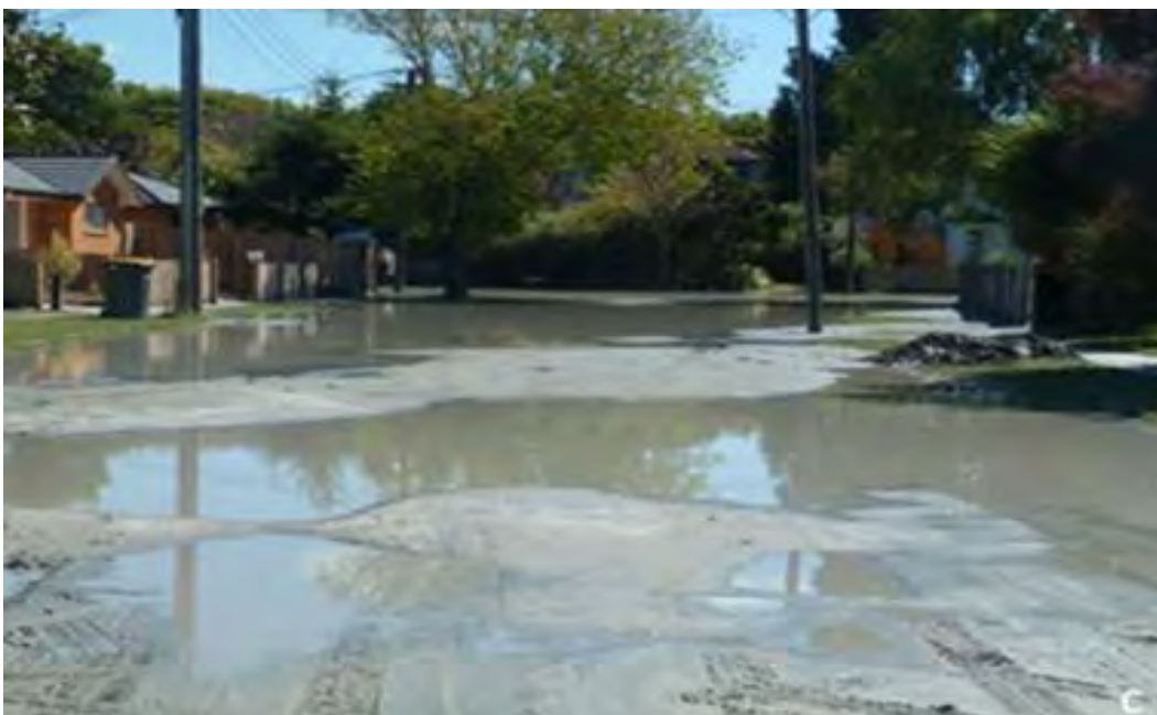
Figure B11 - Photo showing liquefaction in Christchurch following the 2011 Christchurch earthquake. Approximately 200mm to 300mm of liquefaction ejecta inundated the roads.
