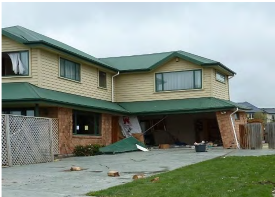
Figure B7 - Photo showing lateral spreading effects at Courtenay Drive, Kaiapoi following the 2010 Darfield earthquake. The total lateral spreading at this site was approximately 2m. If the lateral spreading at the site had been higher, this building would likely have collapsed.
