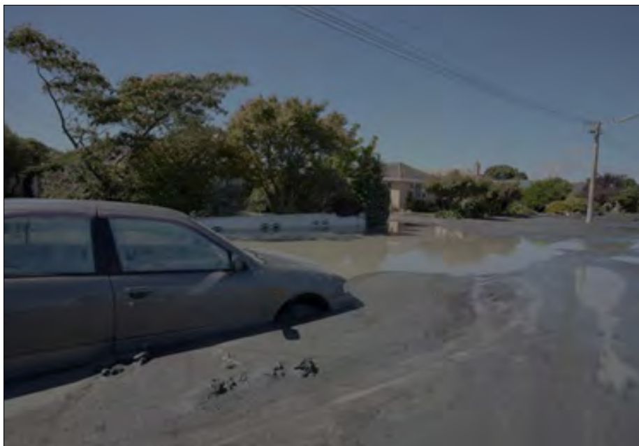
Figure 7: Example of liquefaction following the 2011 Christchurch earthquake, showing the type of liquefaction land damage expected where the LSN is 25 or greater.
