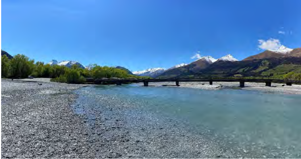
Photo of Rees River bridge, highlighting very limited capacity / freeboard available
