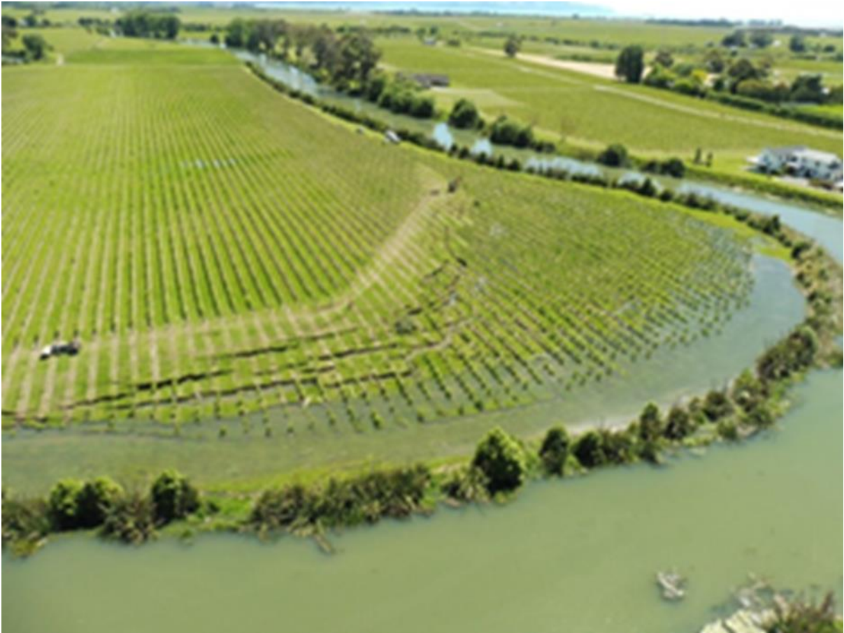
Figure B3 – Photo showing the lateral spreading that occurred in Blenheim at a vineyard along the Wairau River following the 2016 Kaikoura earthquake. The lateral spreading horizontal movement was approximately 3m and the vertical drop was approximately 1m (approx. 33% of the horizontal movement).
