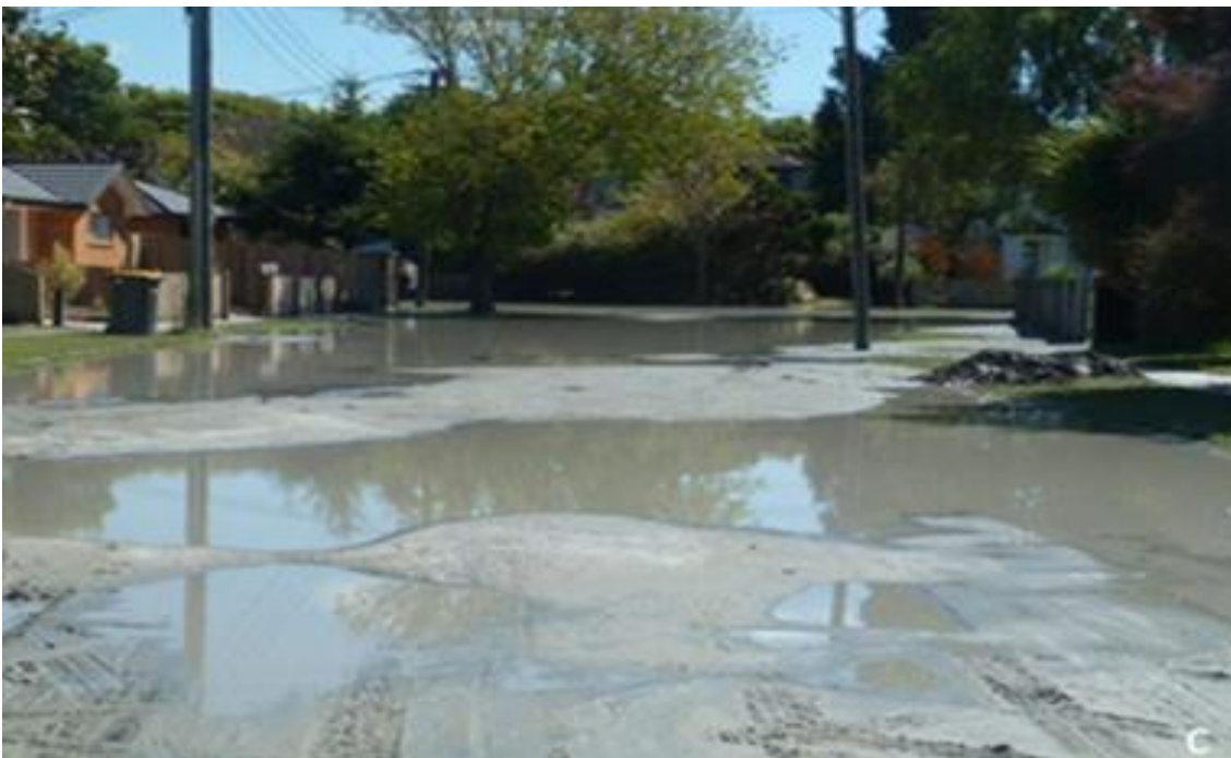
Figure B11 - Photo showing liquefaction in Christchurch following the 2011 Christchurch earthquake. Approximately 200mm to 300mm of liquefaction ejecta inundated the roads.
