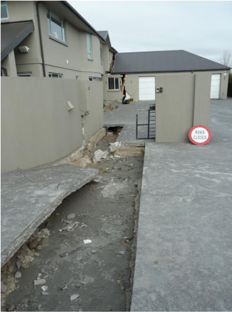
Figure B4 - Photo showing lateral spreading effects at Courtenay Drive, Kaiapoi following the 2010 Darfield earthquake. The ground crack filled up with liquefied sand and resulted in a significant evacuation hazard following the event. The lateral spreading at this site was approximately 2m.
