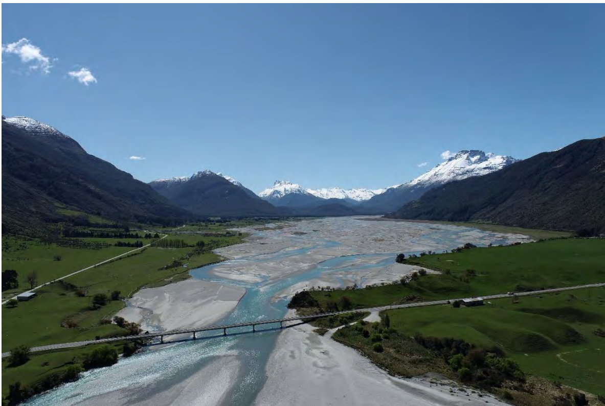
Drone photo of the Dart River bridge (upstream extent of the model)
