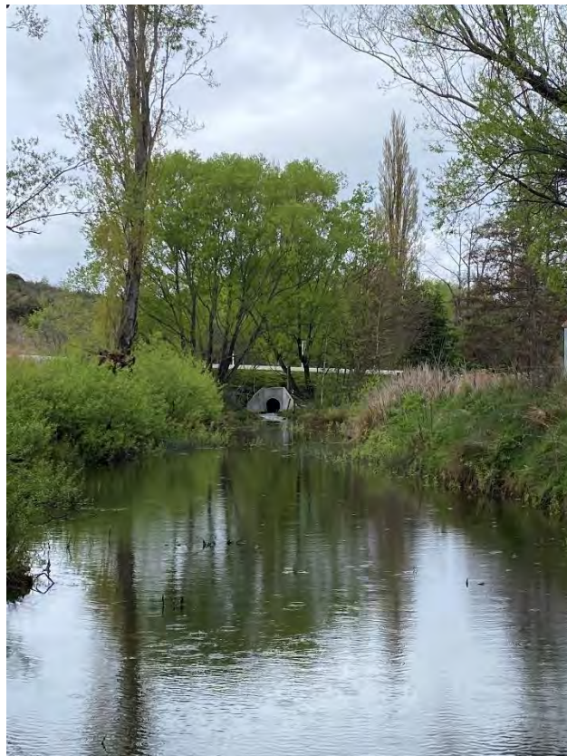
View of culvert under Glenorchy-Paradise Road
