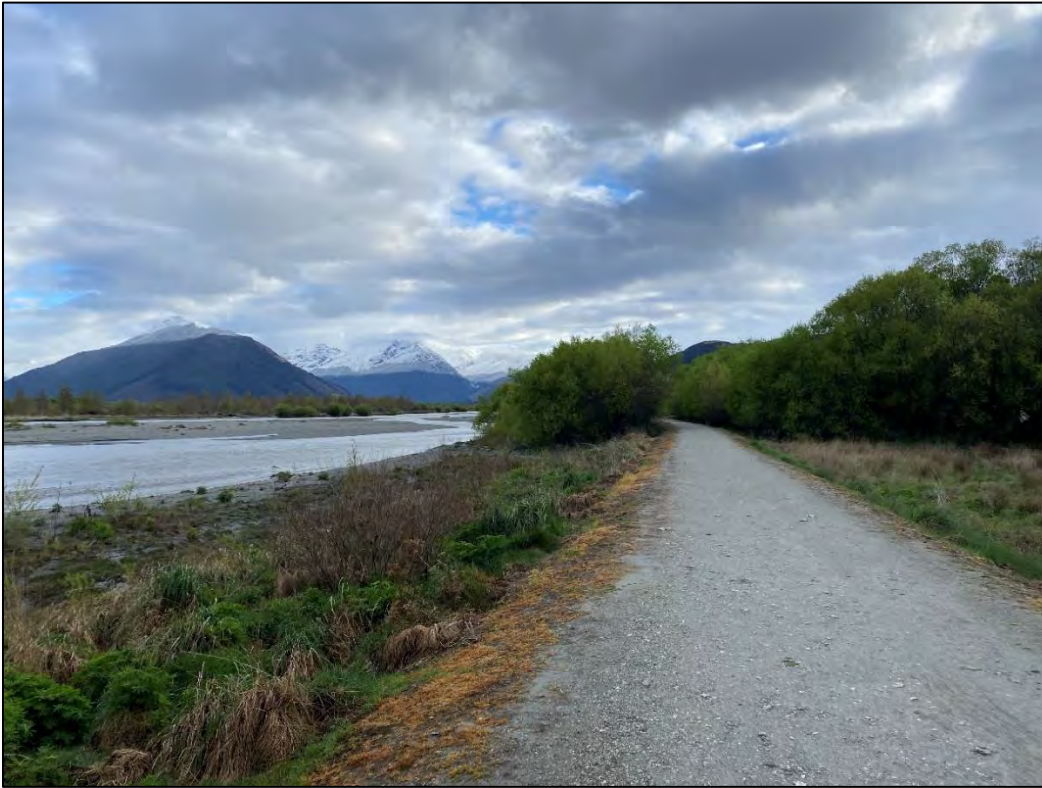
View of Glenorchy Stopbank with Rees River on left
