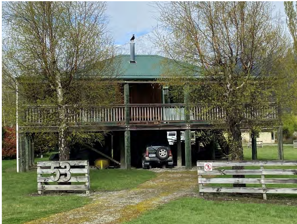
Example of house built on overflow path on stilts (section was significantly flooded in Feb 2021)
