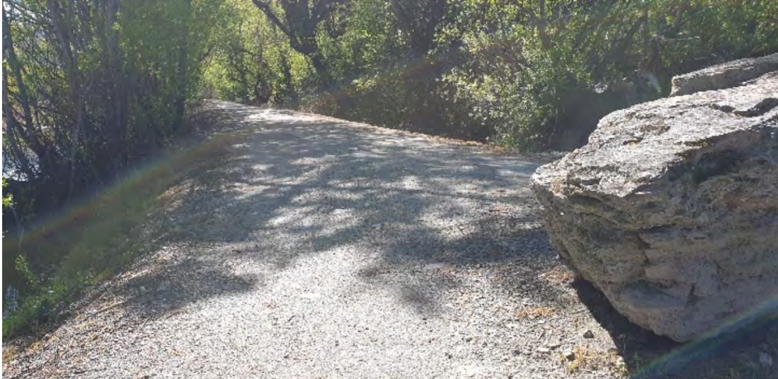
Figure 10 Embankment at location where culvert crosses under embankment. Potential area of interest for piping.
