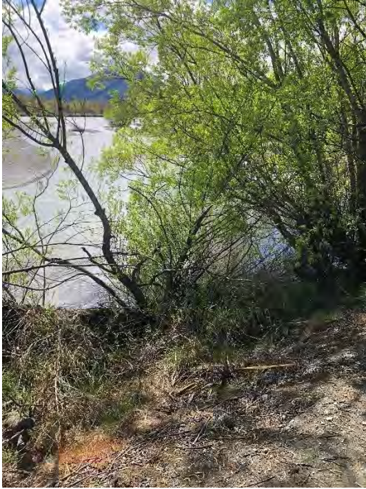
Figure 5 Rees River directed towards the Rees-Glenorchy Floodbank.
