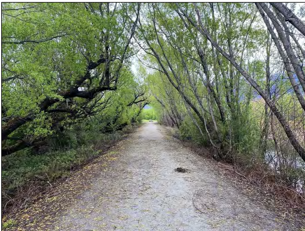
View of Glenorchy Stopbank with Lagoon Creek visible on the right through the willows
