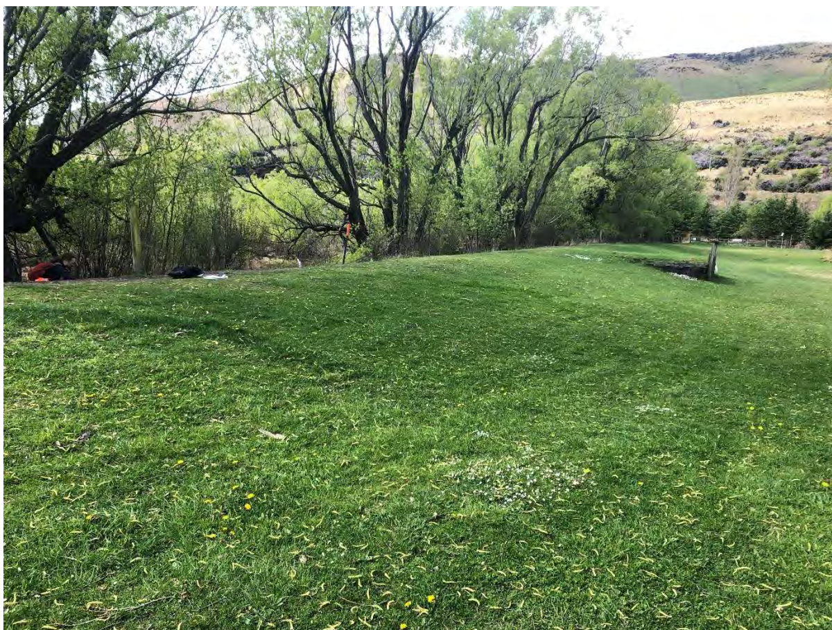
Figure 2 Golf course adjacent to the Rees-Glenorchy Floodbank where sheet flow overtopping has been reported.
