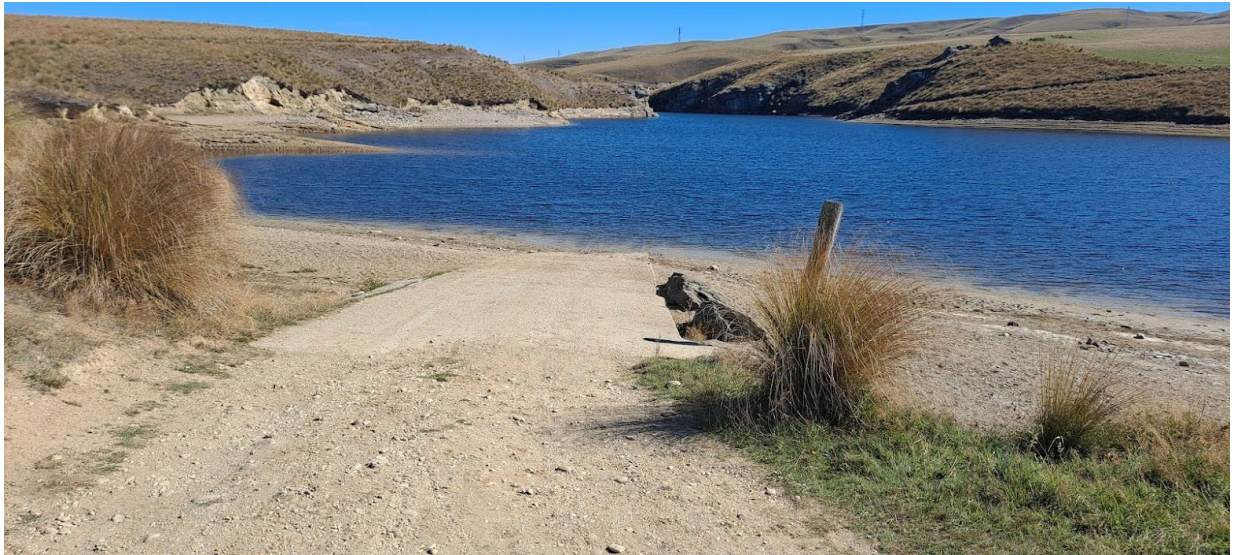
Photo 3: Boat ramp below fishing huts – looking towards dam
