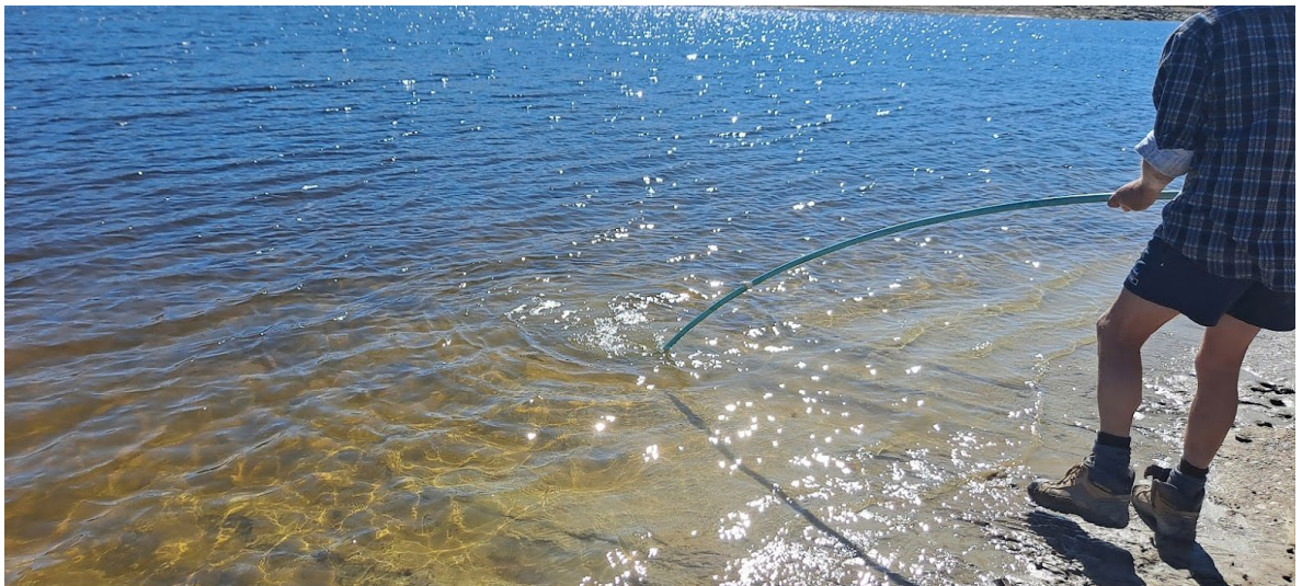
Photo 6: Point where boat ramp ends – shown by pipe
