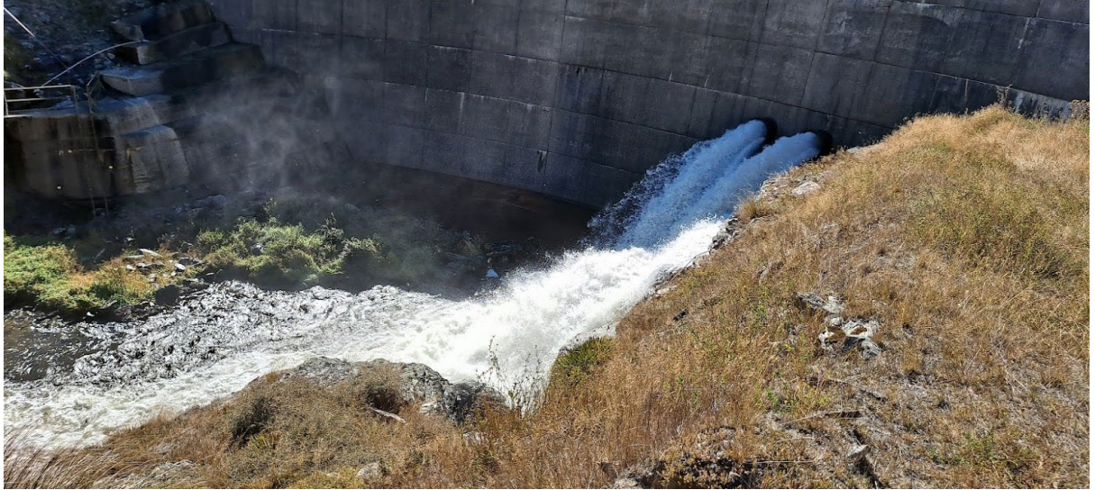
Photo 24: Discharge from Lake Onslow to Teviot River
