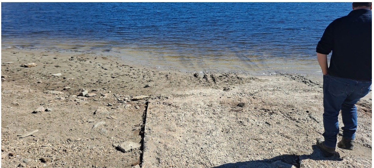
Photo 4: Boat ramp at lake water intersection
