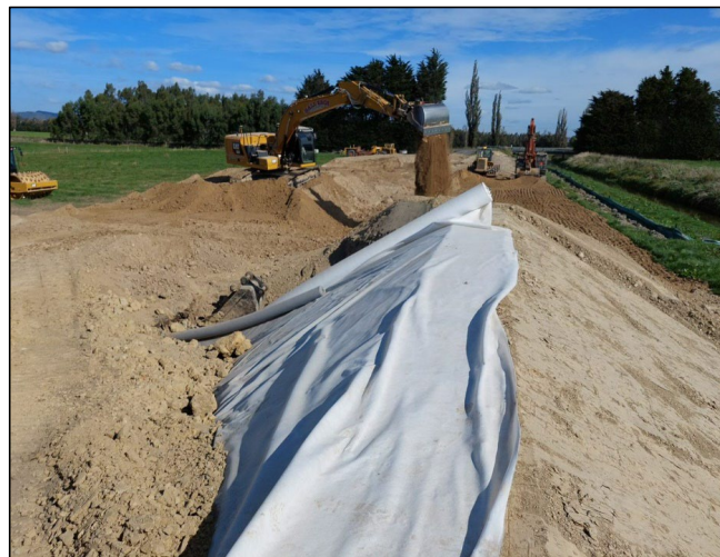
Figure 3. The insertion of geotextile fabric ensure ongoing stability of floodbank.
