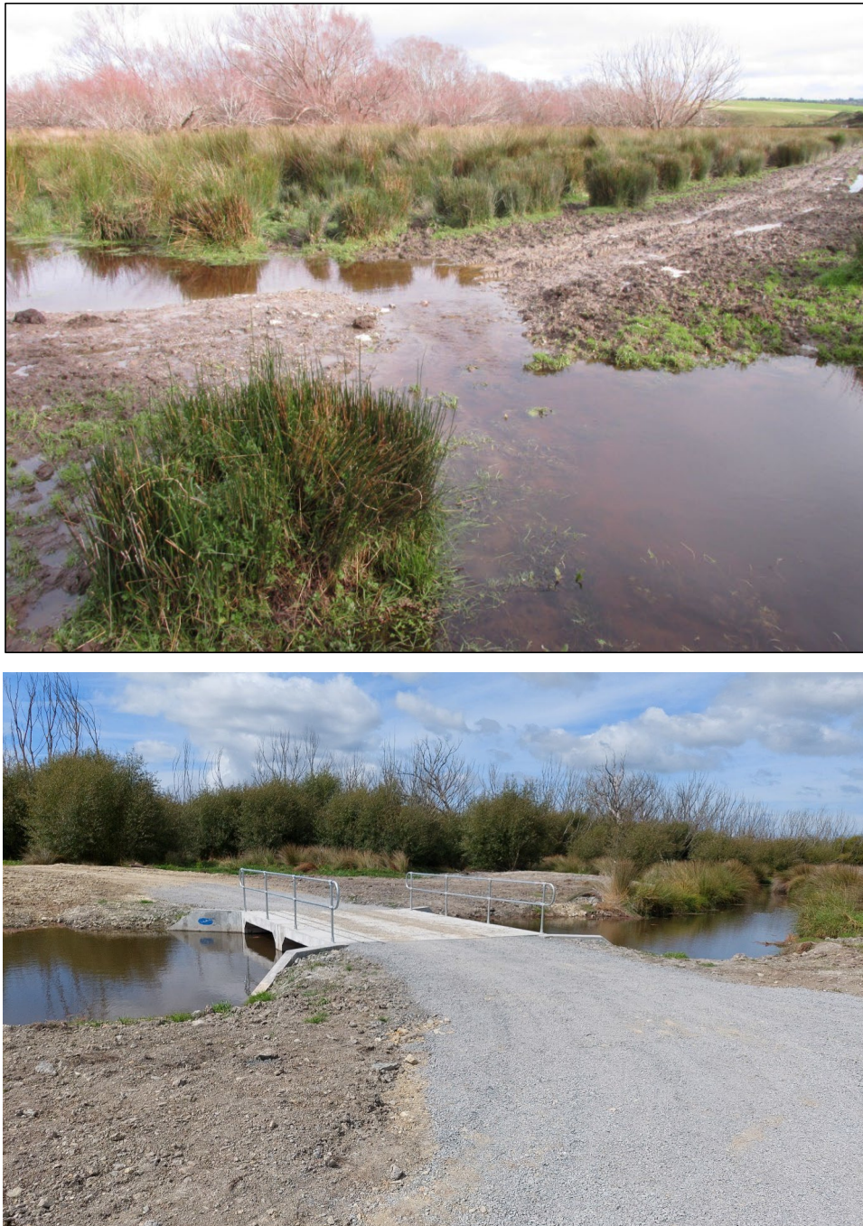
Figure 3. Crossing culvert, before upgrade (upper) and at completion (lower).
