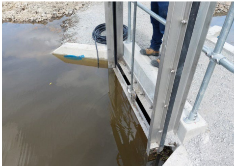
Figure 2: Newly installed structure.
