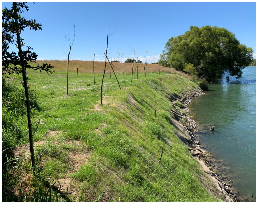
Figure 3. Riverbank Road (262 or LC18) floodbank before(above) and after (below) reshaping and vegetation stabilisation.
