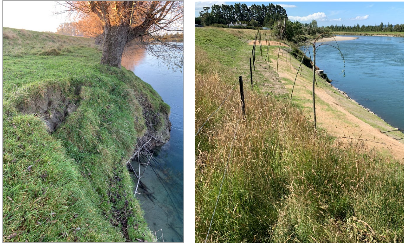
Figure 4. Riverbank Road floodbank at Lawsons (LC20), before(left) and after (right) reshaping and vegetation stabilisation.
