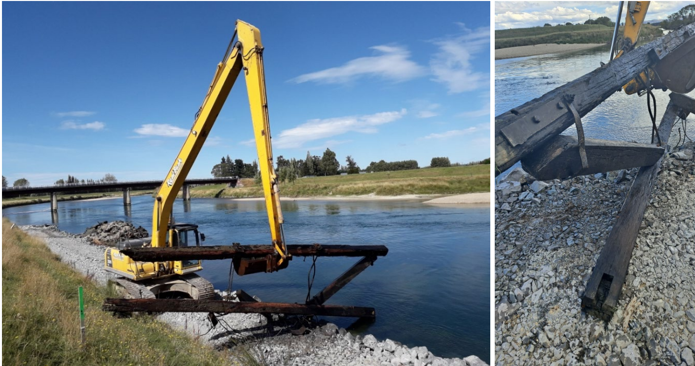
Figure 6. Discovery of historic (Pre-1900) bridge beams at Riverbank Road floodbank works at bridge near Stirling (LC21).
