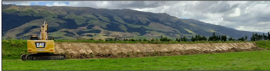
Figure 2. Topsoil being removed during the deconstruction of stage 5.
