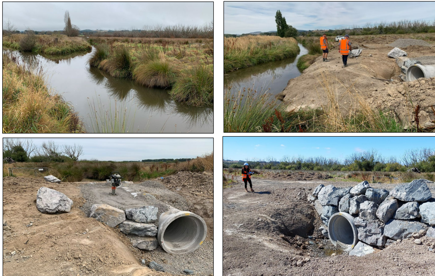
Figure 4. Flow culverts, before upgrade, during works and on completion.
