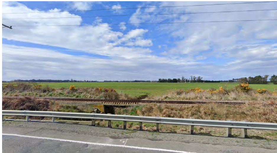
Figure 6: Hilderthorpe Floodway; view east from State highway 1 bridge.
