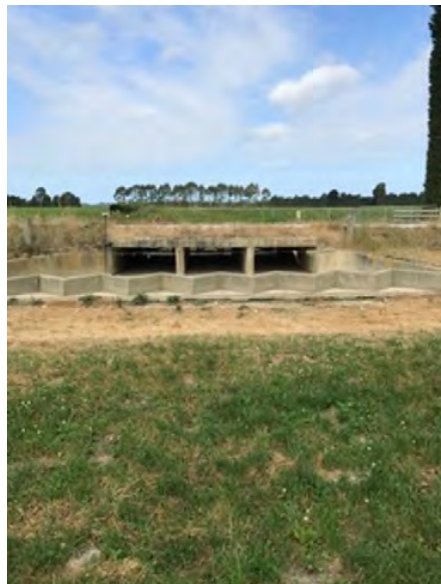
Figure 8: Western view of the Hilderthorpe Floodway Gray Road crossing
