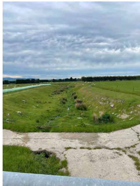
Figure 11 Waikoura Creek Floodway, viewed from State highway 83 towards the north east.
