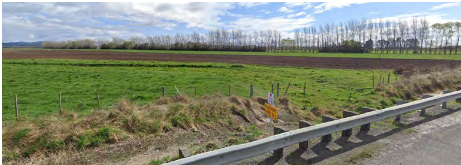
Figure 1: Hilderthorpe Floodway at State highway 1 (source: Google Streetview)
