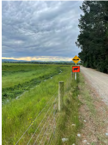
Figure 14: Henderson and Waikoura Creeks Floodway; viewed from opposite 550 Jardine Road, looking towards the north.
