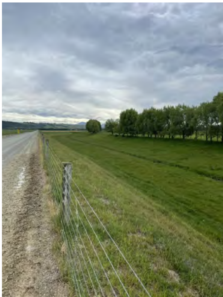
Figure 10: Henderson/Waikoura Floodway from Irvine Road (upstream)
