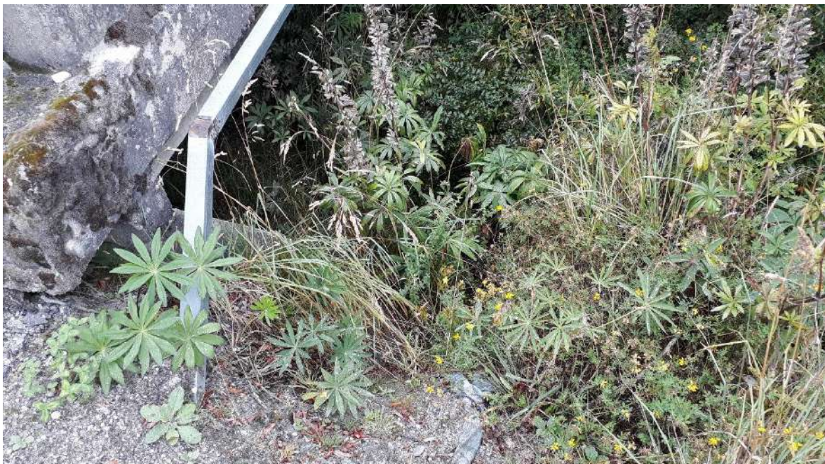
Figure 6.4: View under right abutment of Rees Bridge from downstream side of road embankment
