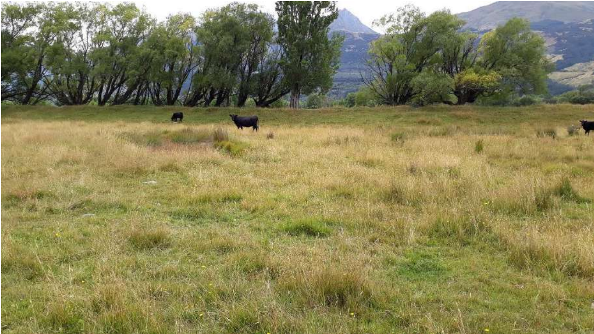
Figure 6.6: Secondary stopbank on right bank upstream of Rees Bridge which runs parallel with Paradise Road
