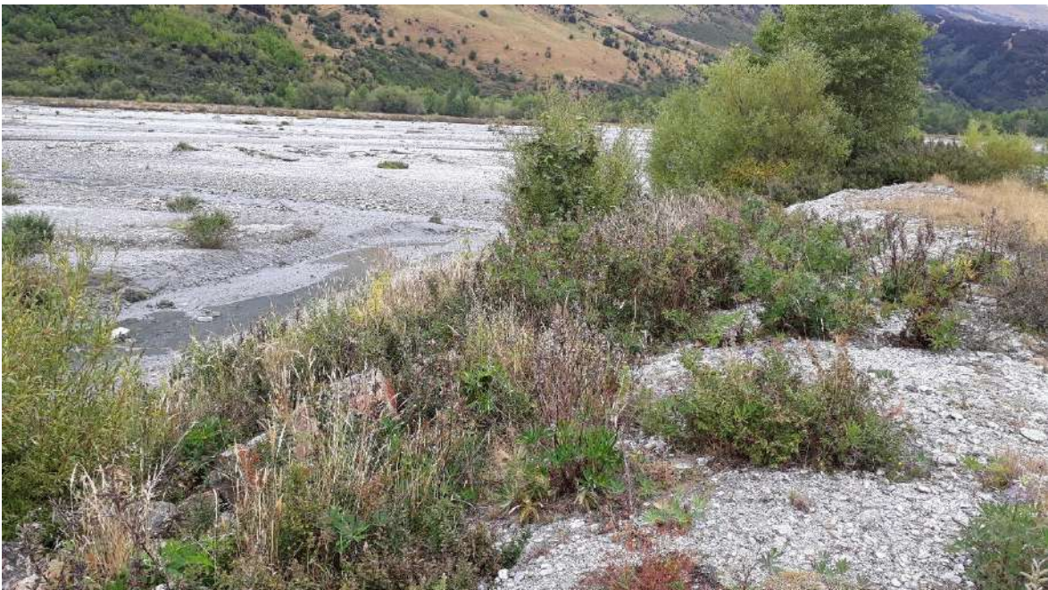
Figure 6.7: Rock groyne structure on right bank of Rees River upstream of existing bridge (the head of the structure beyond the willow saplings in the right of the photo was damaged in a recent flood event)
