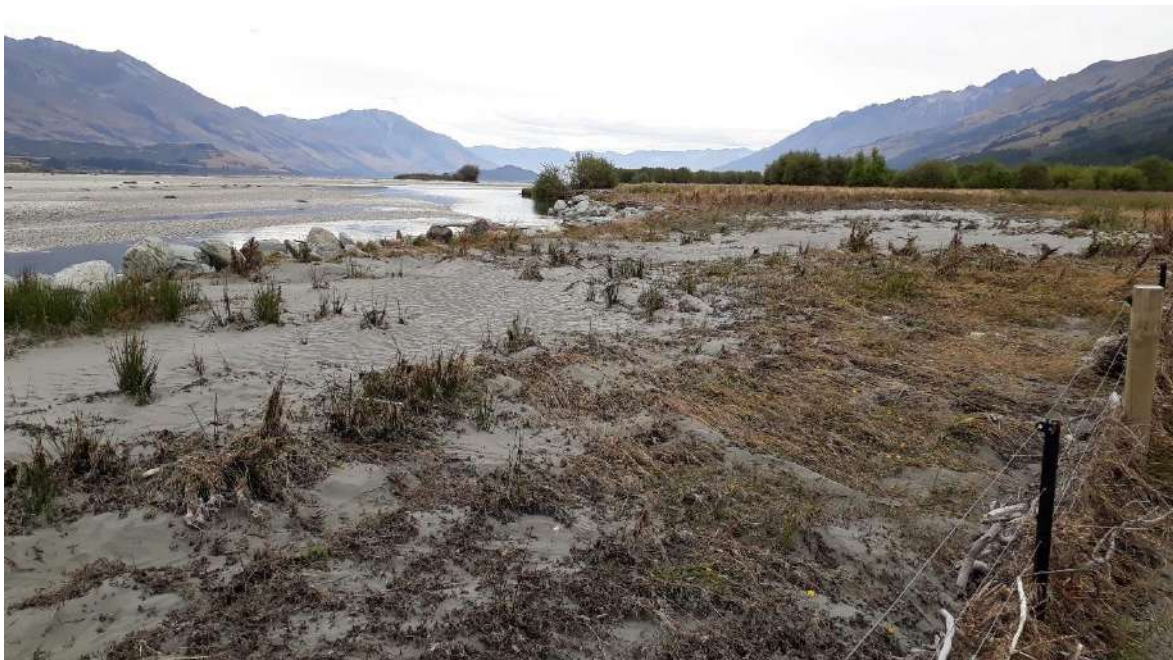
Figure 2.5: Erosion protection works adjacent to Kinloch Road with evidence of recent breakout flows across road in February 2022 (note level of riverbed adjacent to right bank floodplain)
