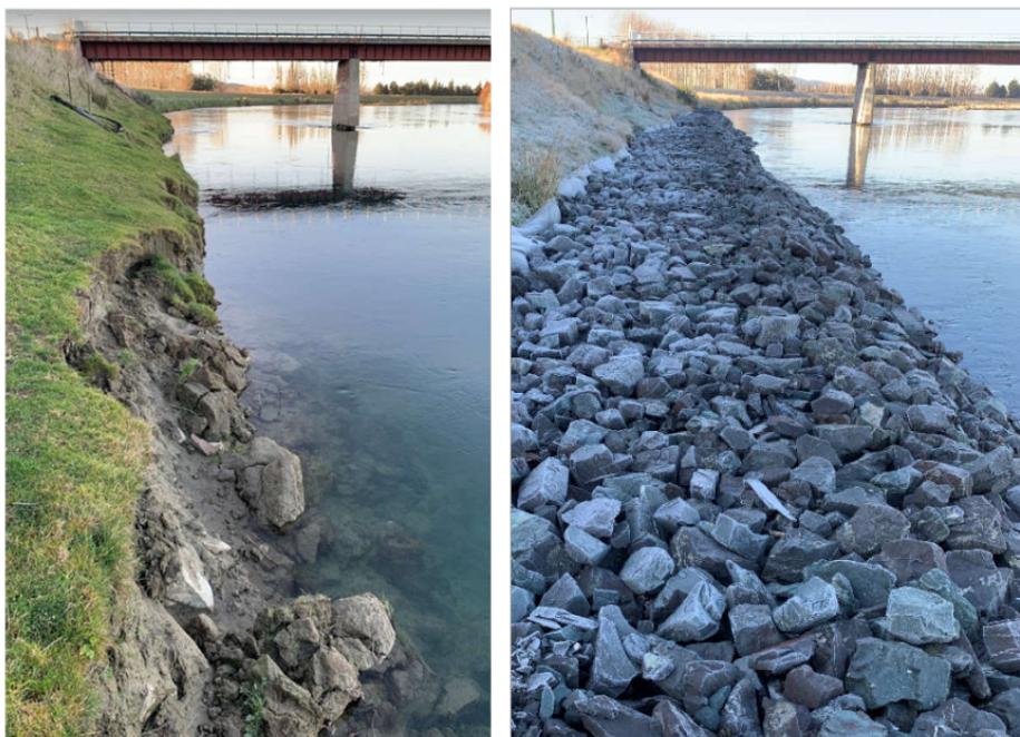
Site LC21, Riverbank stabilisation before (left) and after (right)
