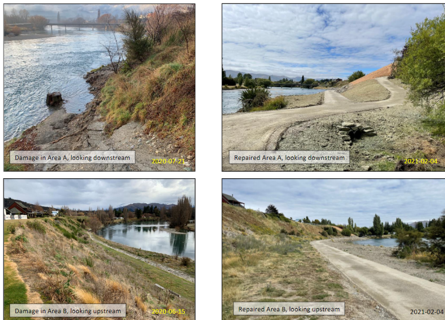
Riverbank stabilisation before (left) and after (right)
