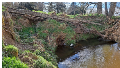
Tokomariro River, West Branch, 300m upstream from SH Bridge
