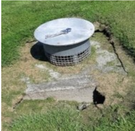
Photo 6 (L) and 7 (R); Relief Well #34 showing subsidence and Relief Well #7 showing offset in pipe joint.
