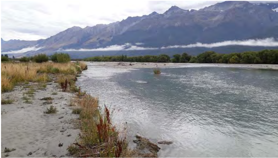
Figure 2.9: View looking downstream along the left bank of the Lower Rees River showing evidence of loss of freeboard and sediment deposition from recent flood breakout flows (photo taken on 9 February 2022 near start of bed level change map in Figure 2.8 – river flow \approx 13 \text{ m}^3/\text{s} at time of photograph)
