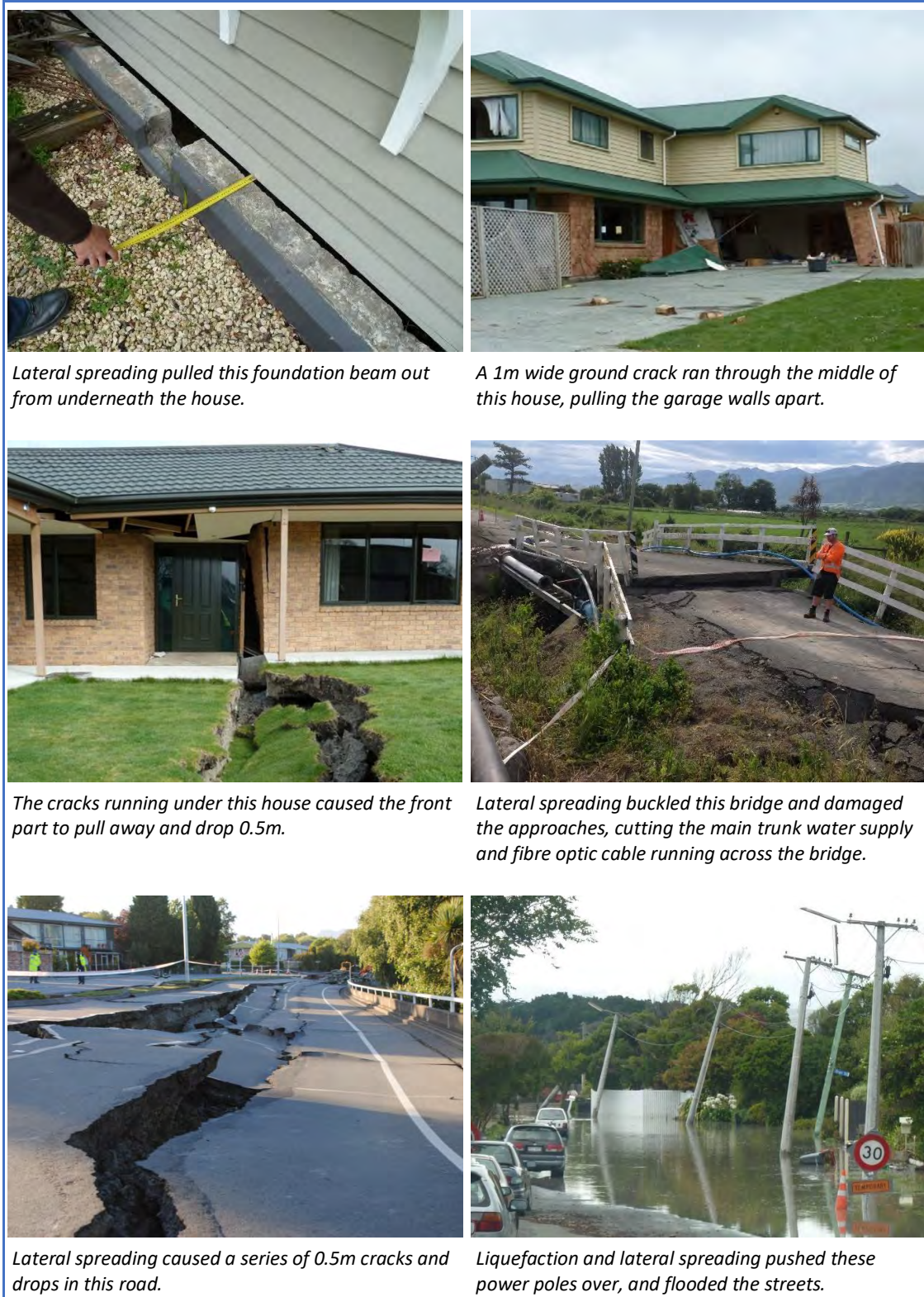
Figure 2.3: Example photographs of the types of damage to land, buildings and infrastructure that could be expected in a large earthquake in the parts of Glenorchy categorised as Major and Severe lateral spreading. For these examples the free face was about 4m high. In Glenorchy the free face is much higher (about 25m below lake level), so lateral spreading could be more severe and extend further inland.
