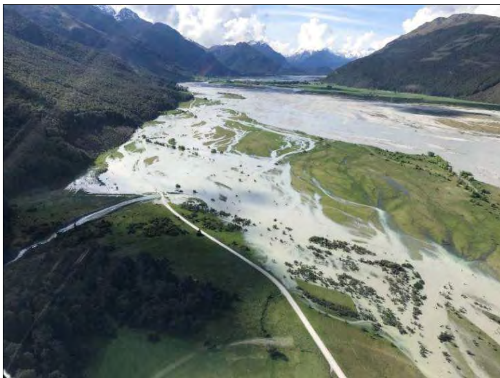
Figure 2.4: Flooding of Kinloch Road (in the foreground) in a minor flood event in 2019 - Dart River floodplain looking upstream
