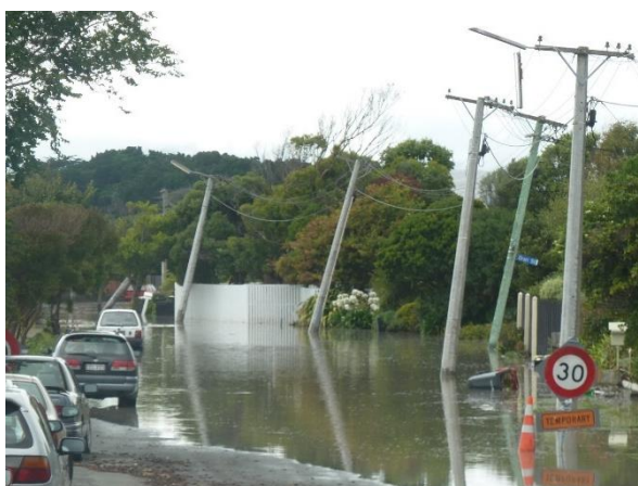
Liquefaction and lateral spreading pushed these power poles over, and flooded the streets.
