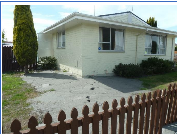
Liquefied sand ejected from underneath a house.
