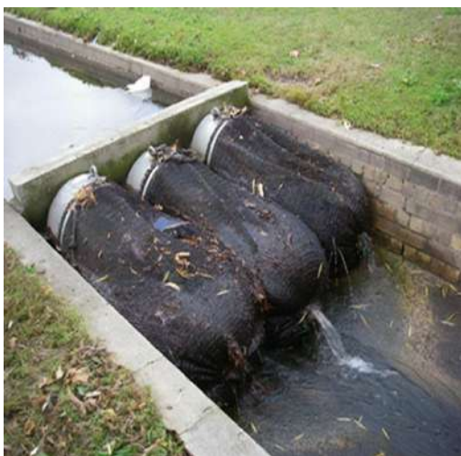
Figures 3&4 show the type of stormwater filters utilised in removing plastics that enter in significant waterways like the Otago Harbour.
