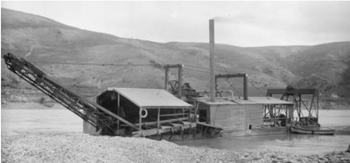
Figure 16 – Golden Treasure dredge just prior to sinking
