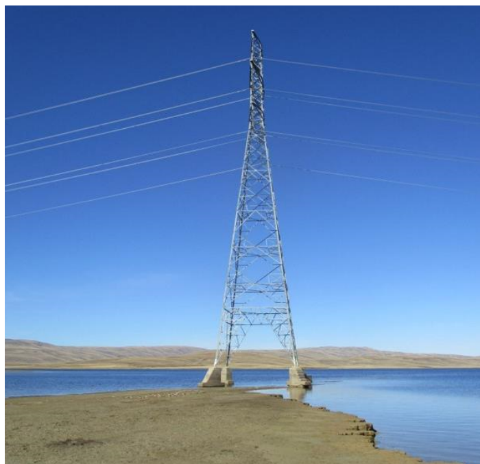
Figure 1: Tower at Lake Onslow
