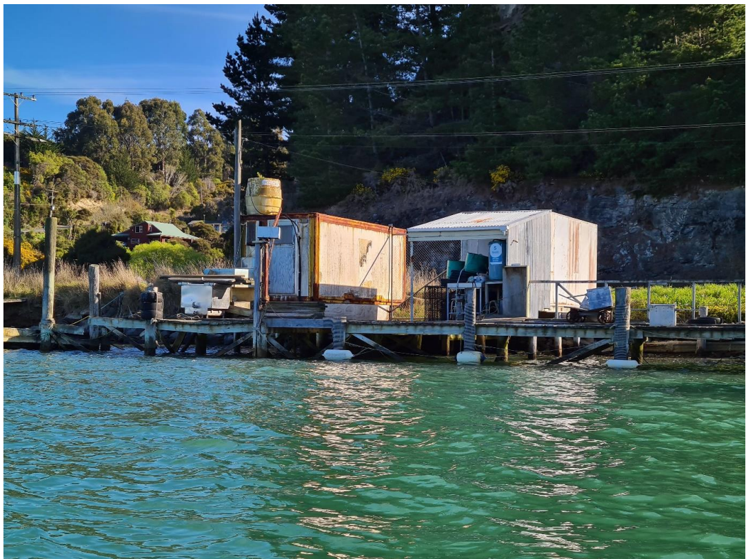
The existing structures, which have been recently tidied up somewhat by the applicant
