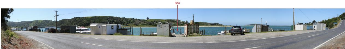
Figure 8 View of site from the west. Source: Moore, 2023.
