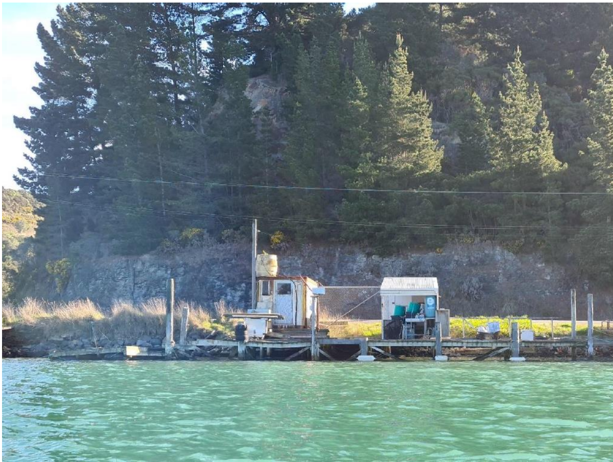
Figure 4 Photograph of current structures from the CMA. Source: RM22.550 application.
