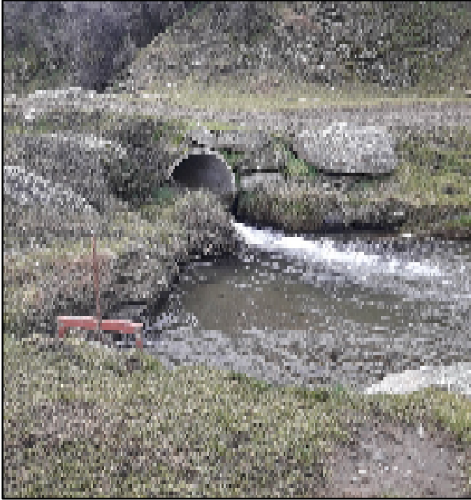
Figure 3: Sluice gate intake at Matakanui culvert crossing over Neds Creek (August 2018)
