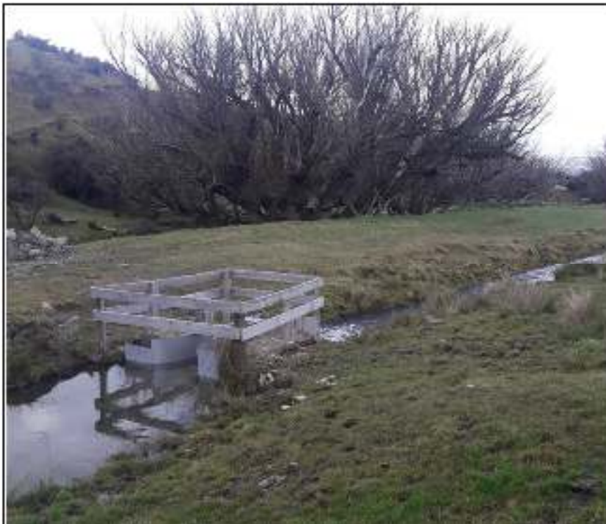
Figure 7: Water measuring station on water race (August 2018).
