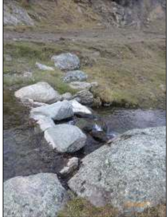
Figure 4: Rock embankment below intake sluice gate (2015)
