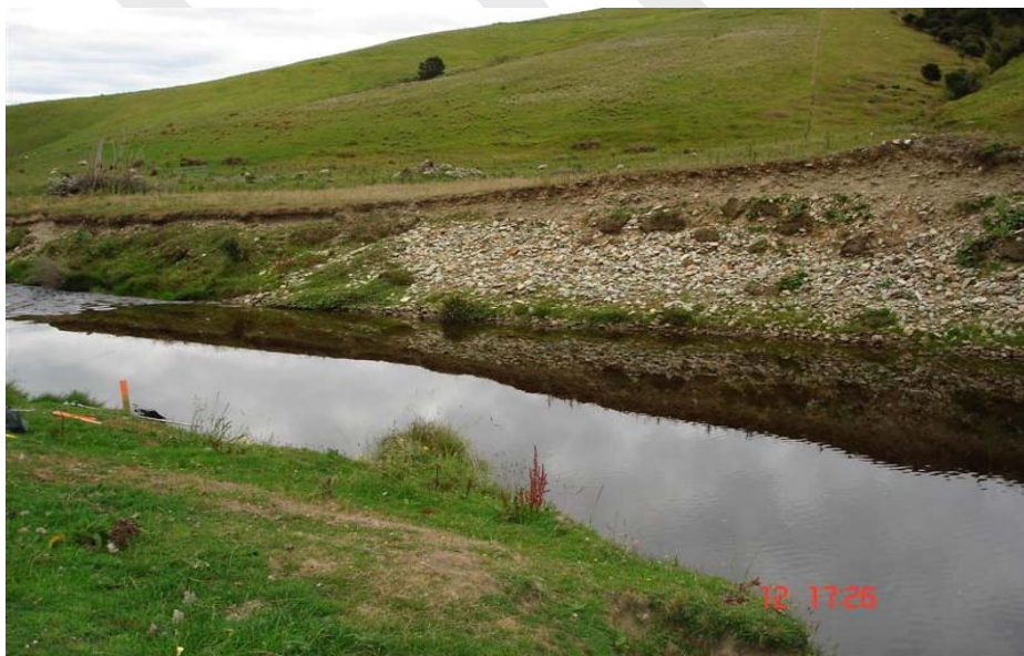
Figure 4: Upper Waitahuna River gauging site (cross section 15)
