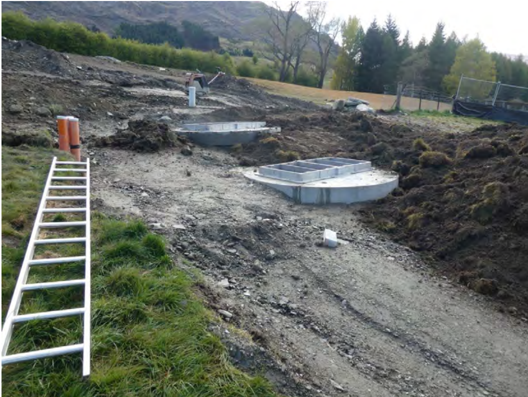
Figure 8: Mill Creek (Arrow River water) augmentation works under construction.
