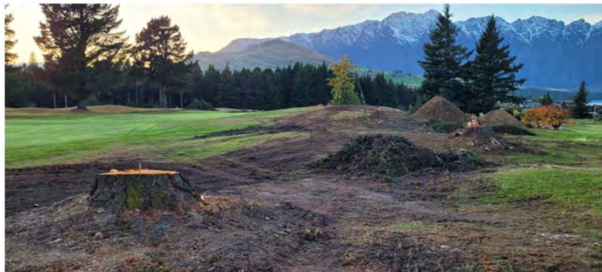
Clean up on site has been supported by the Queenstown Golf club grounds staff and an army of golf member volunteers. A plentiful volume of chips has also be produced which will help the club with its replanting plans
