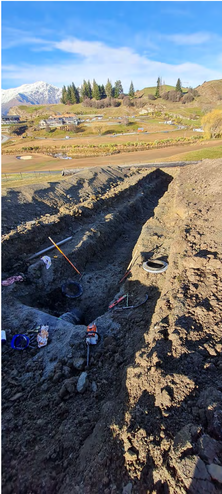
Figure 7: Mill Creek (Arrow River water) augmentation works under construction, pipe trench.
