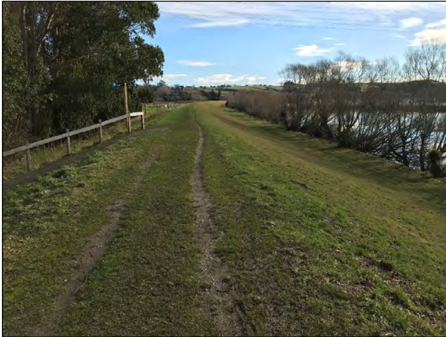
Figure 5: Example of ORC flood banks in the Balclutha township area, showing the scale of these flood protection structures. This location is upstream of the SH1 bridge.
