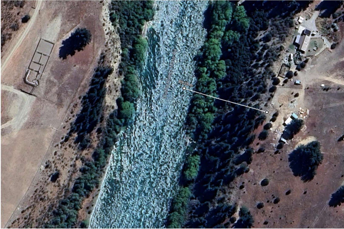
D - Māori Point Road – Approx 90 metres
