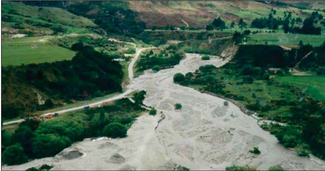
Figure 3-5 – The Buckler Burn following the November 1999 flood event, showing debris deposition over the Queenstown-Glenorchy Road on the true right bank.
