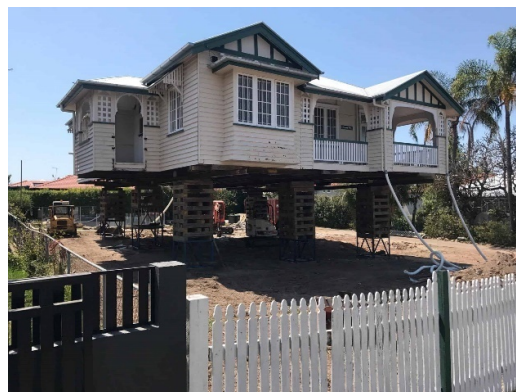
Figure 2.1: A house that is being raised [6].
