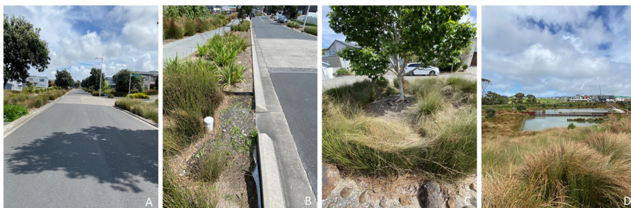
Figure 5.2: Stormwater management features used in Long Bay A. Rain gardens line residential streets B. Rain gardens with mesh and stones C. Garden Street with a large rain garden at the end of a cul-de-sac D. Wetland constructed to retain stormwater runoff.
