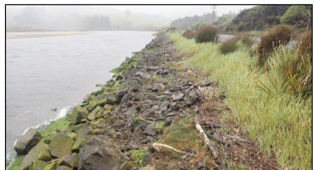
Rock armoring of roadside margin.
